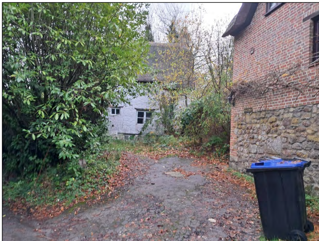
Photo. 12 High View, as viewed from Oak Lane
