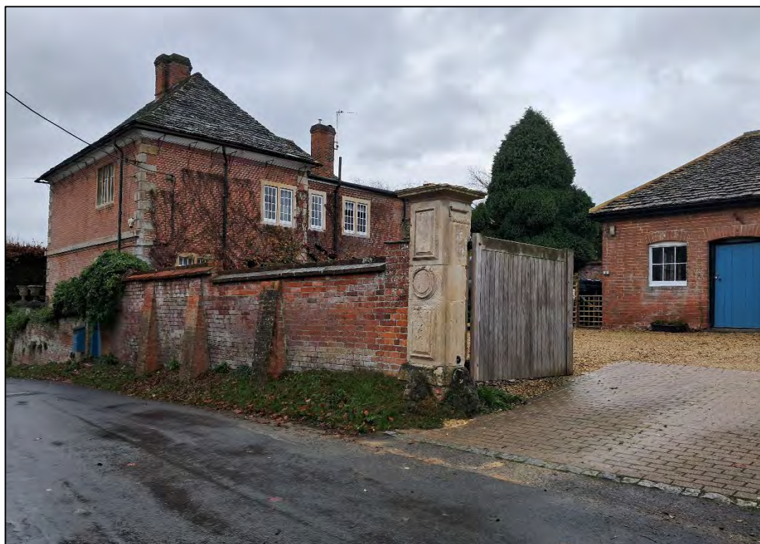
Photo. 9 View of Kestrels and the area to the rear of the Listed Building from Oak Lane
