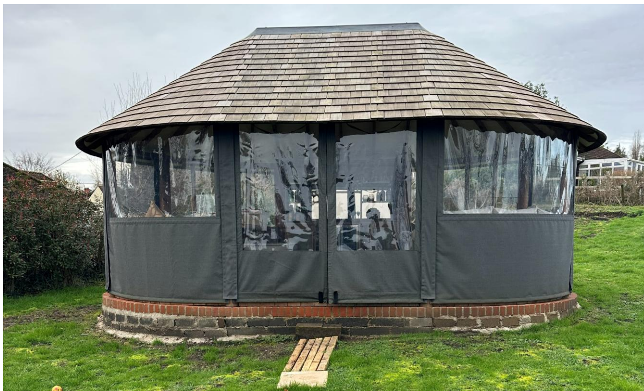
Garden building - north east elevation
