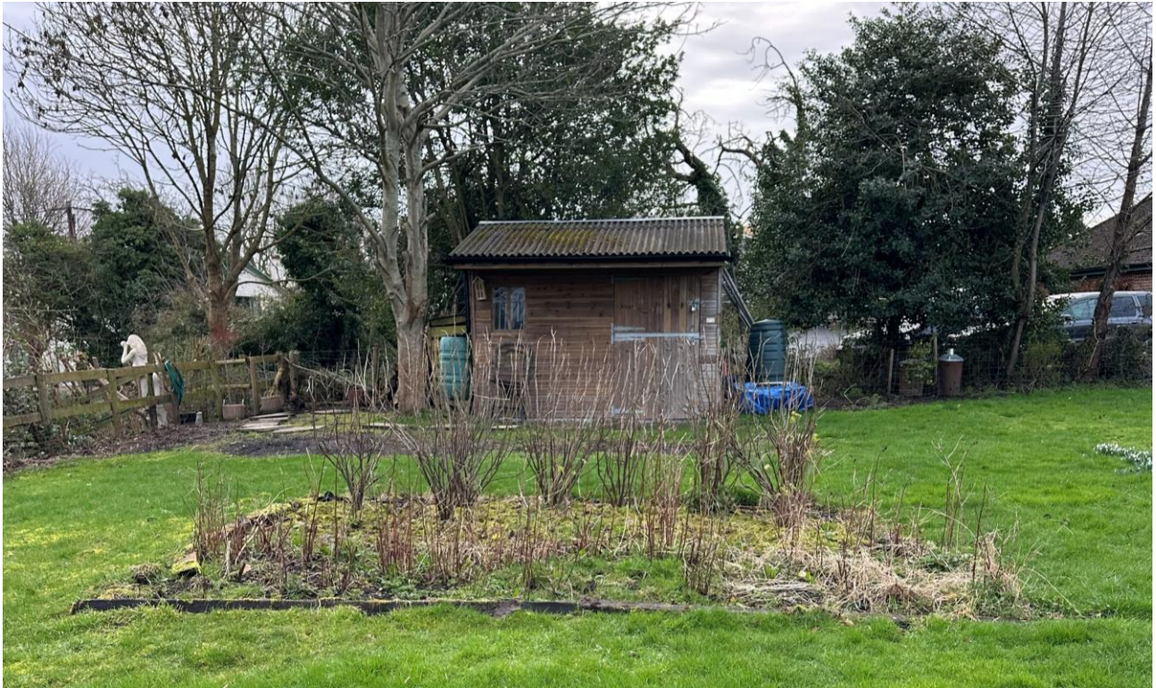
Pre-existing stable building in south east corner
