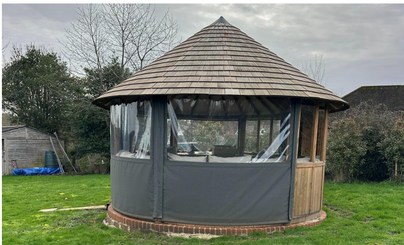
Garden building - north west elevation
