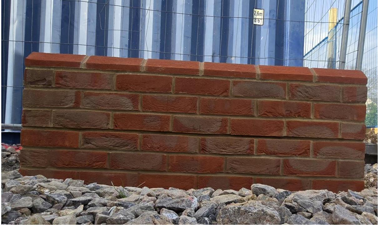
Photo of sample panel on site.
