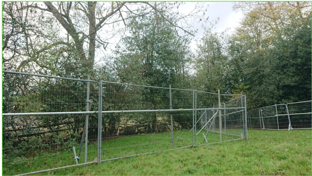
Typical tree protection barrier construction
