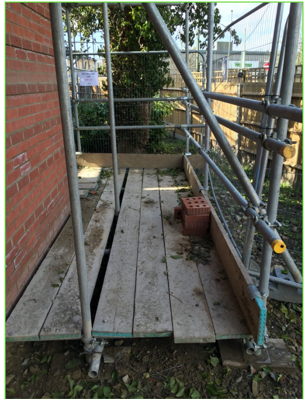
Scaffold ground protection
