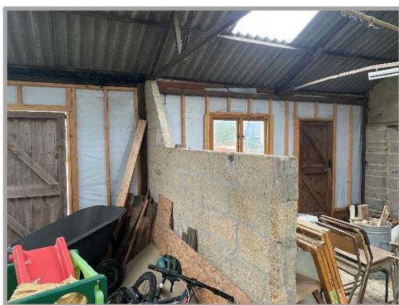
Internal (front wall)
