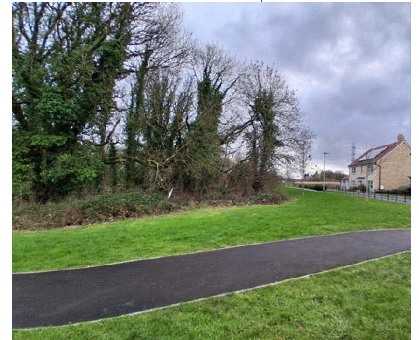
Bitmac footpath 2m wide, with concrete edging
