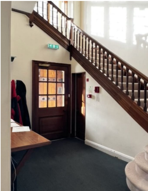
Site Picture of Existing door
