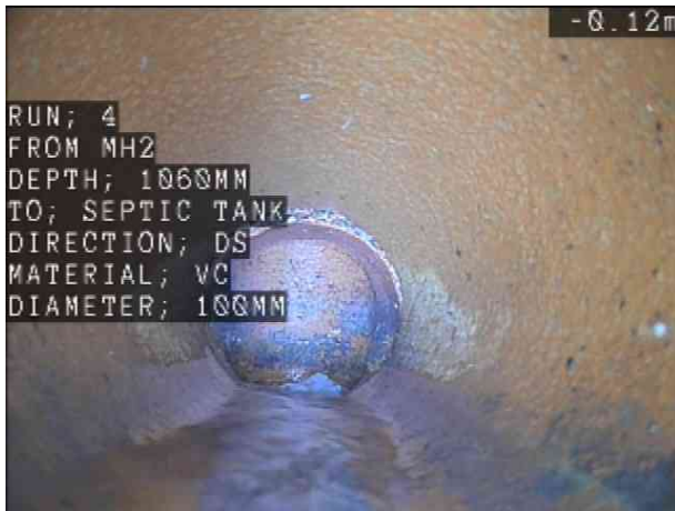
MH2X_a05100ac-8c38-492d-9afd-7886afe9066f_20241206_131116_872.jpg, 00:00:00, 0.00 m Start of survey
