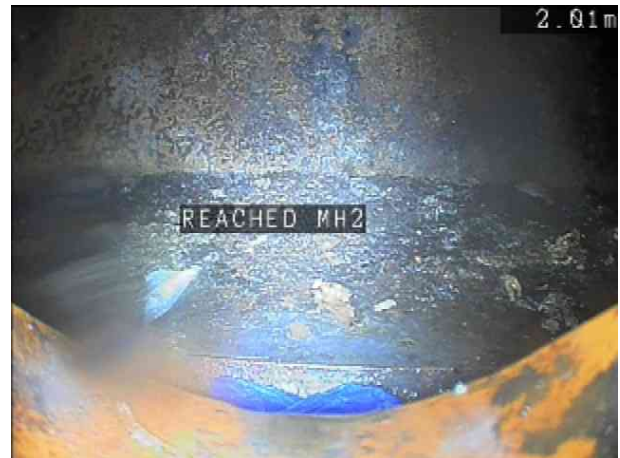
MH3X_dc45c5f1-236d-4b7f-a62d-ae4e1352548_20241206_131546_306.jpg, 00:00:17, 2.01 m Finish survey, Reached MH2
