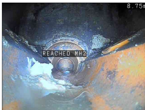
MH1X_c785dc95-92f0-404f-95e0-0695f763a338_20241206_131047_998.jpg, 00:01:02, 8.75 m Finish survey, Reached MH2
