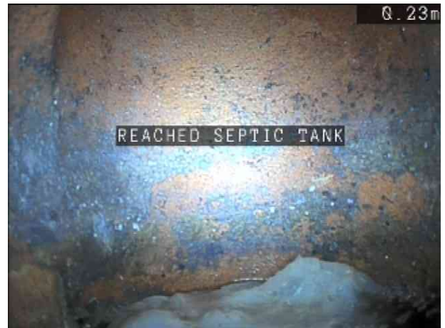
MH2X_1efb10a0-5498-4782-946a-04e523c5b8a2_20241206_131232_254.jpg, 00:00:18, 0.23 m Finish survey, Reached septic tank inlet
