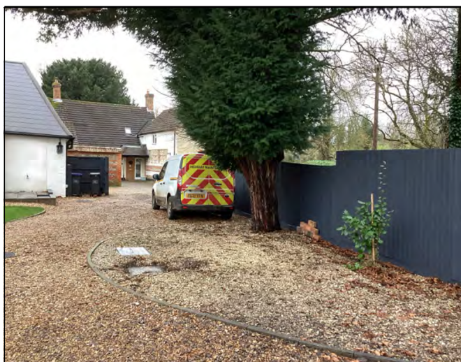
septic tank and the new STP location
