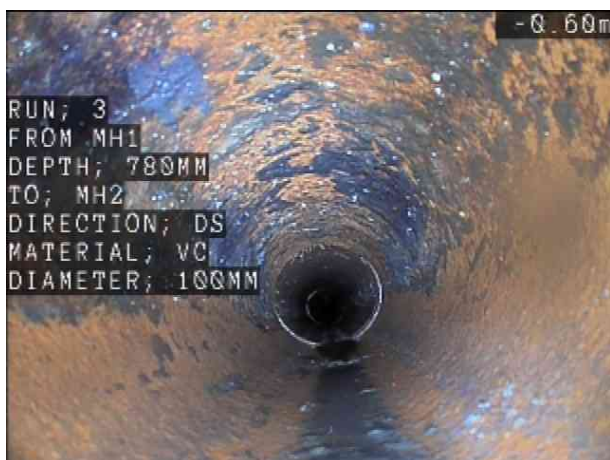
MH1X_f9b0725a-5eb0-4d38-8f2c-04eef8e5a83d_20241206_130728_703.jpg, 00:00:00, 0.00 m Start of survey
