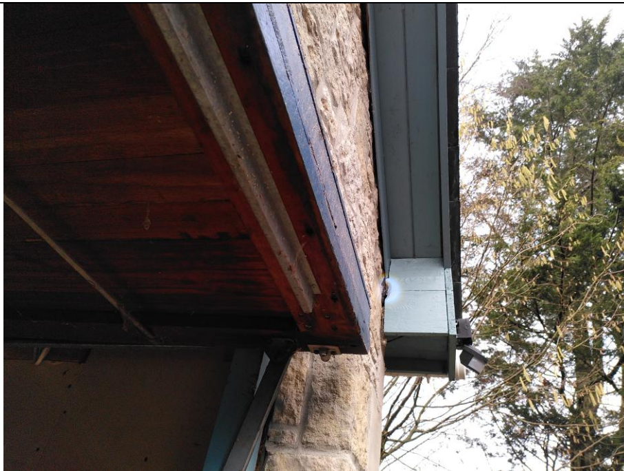
Fig 5. The eastern corner hole appeared to have been gnawed or caused by a knot hole in the board.
