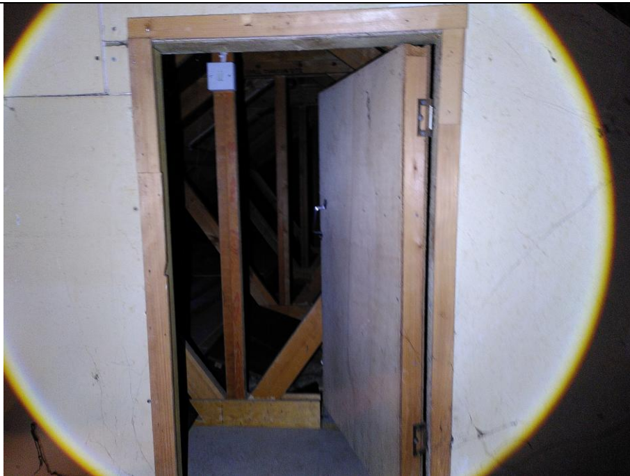
Fig 8. Access door between garage and link roof voids.
