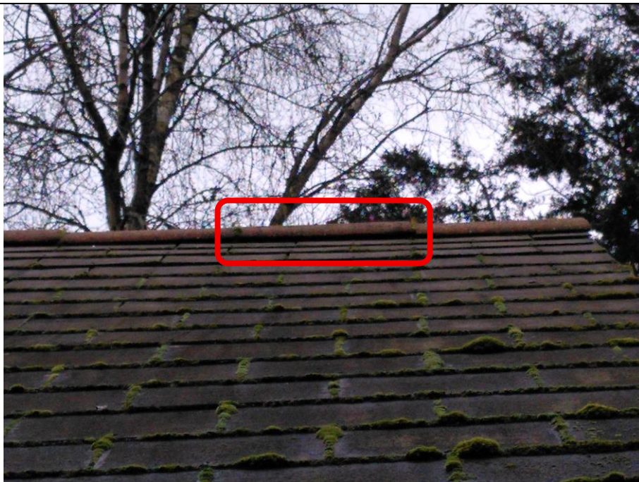
Fig 7. Example of raised ridge tile.
