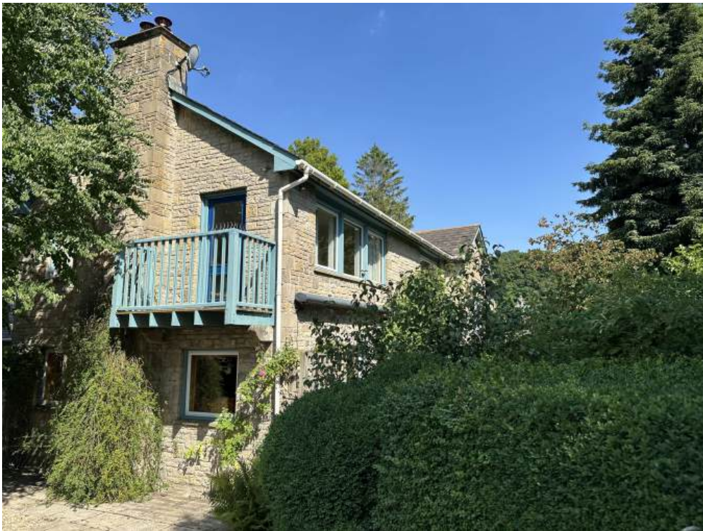
Photograph 02, Existing dwelling from gardens.
