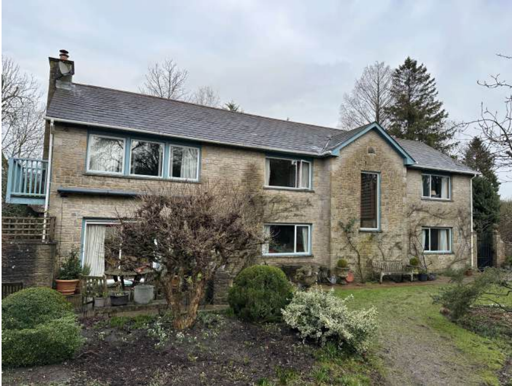
Photograph 05, Existing dwelling from gardens.
