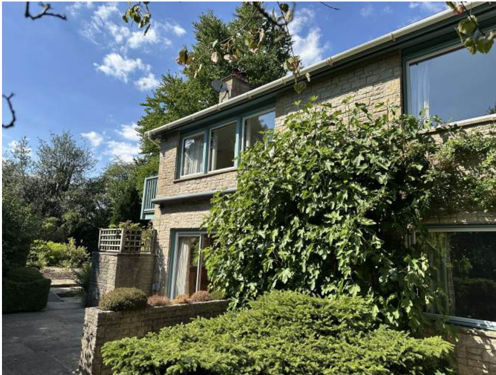
Photograph 03, Existing dwelling from gardens.
