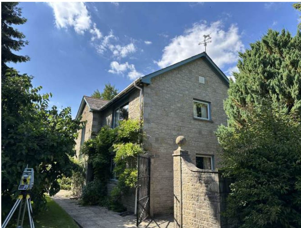
Photograph 04, Existing dwelling from gardens.
