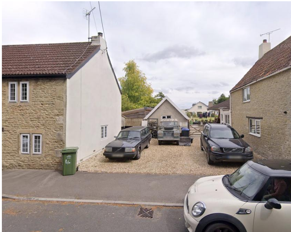
Image of the street scene with the subject outbuilding in the background.
