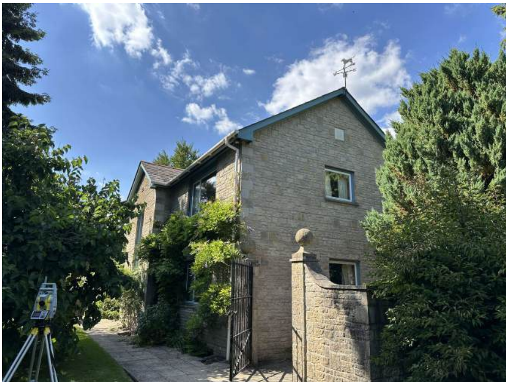
Photograph 04, Existing dwelling from gardens.
