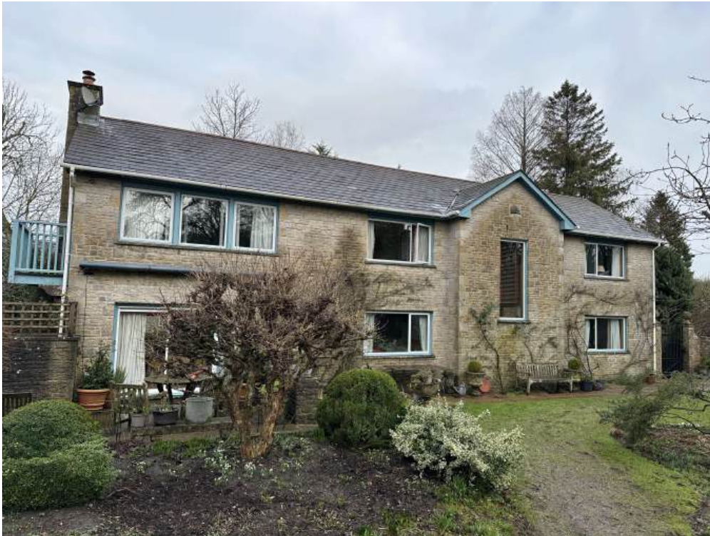
Photograph 05, Existing dwelling from gardens.
