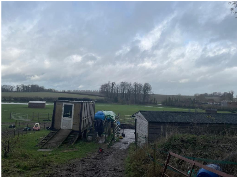
Image 04 – The southern aspect of the proposed new stables and covered yard. Buildings 04 and 06 are partially visible, assessed as offering ‘low’ bat roost suitability.
