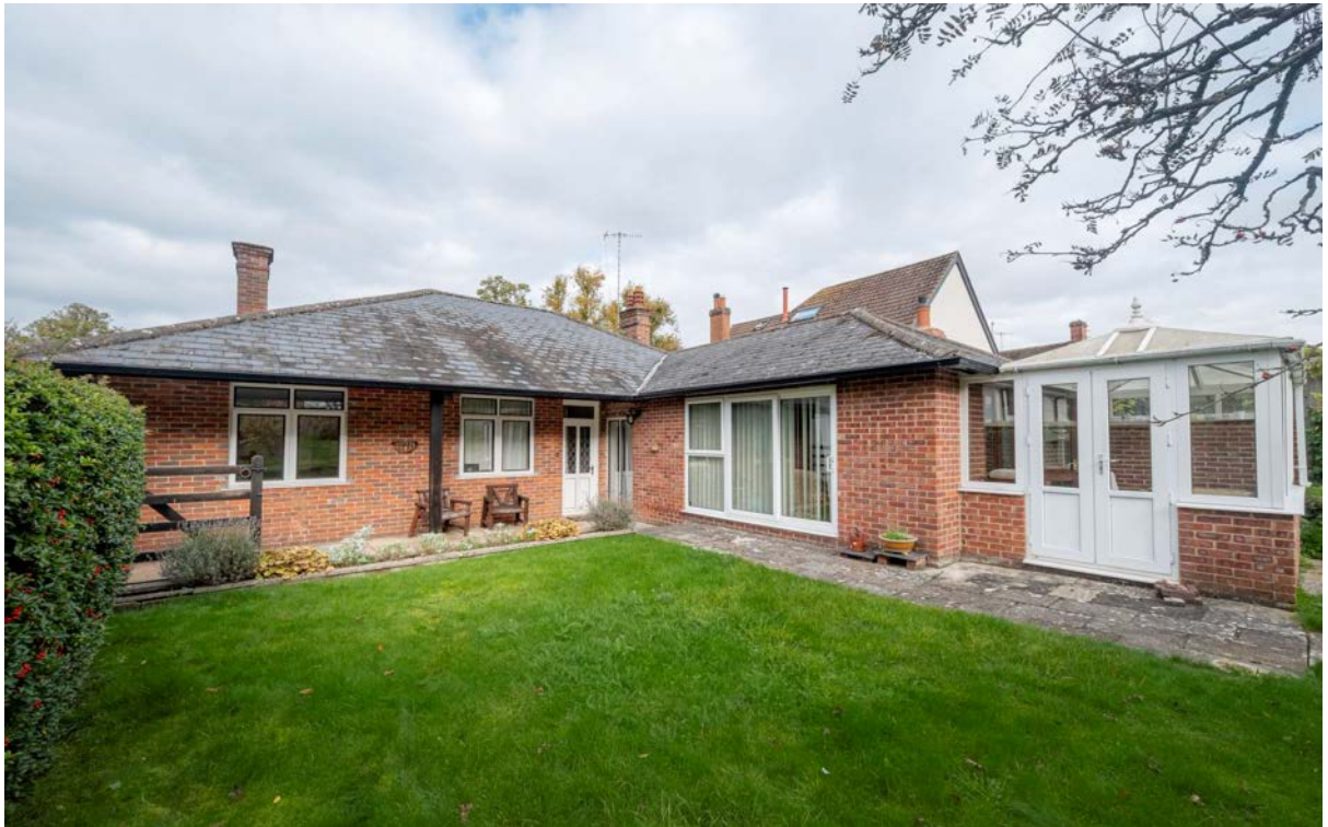
Figure 12: Existing Dwelling from Rear.
