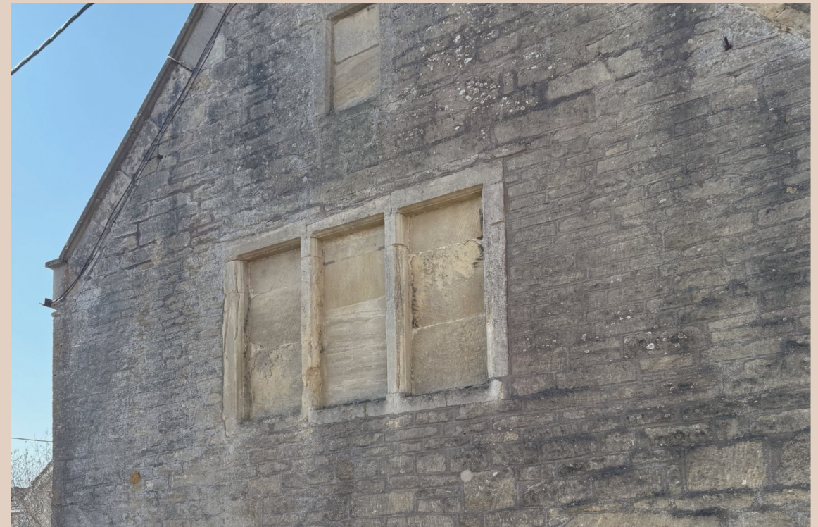
Stone mullioned blank windows on gable end of number 19.
