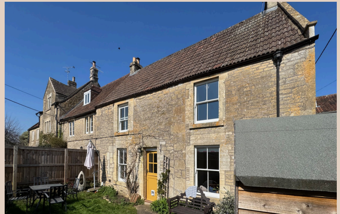
Rear of number 19 showing context of adjoining cottages.
