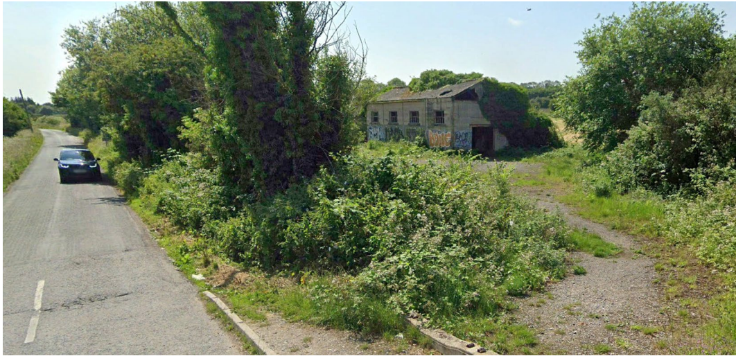
Coate Road: Existing Building in Northwest of the site.
