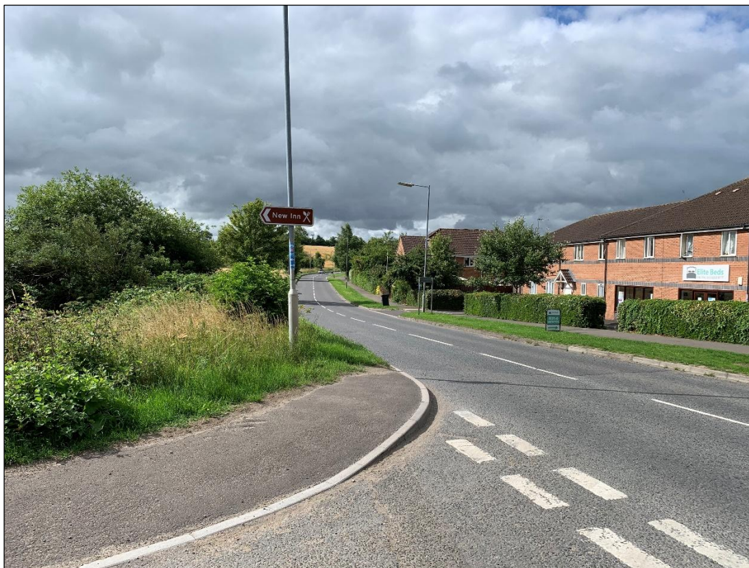
Photograph 3.4: View to the south along Windsor Drive from the Windsor Drive/Coate Road Junction
