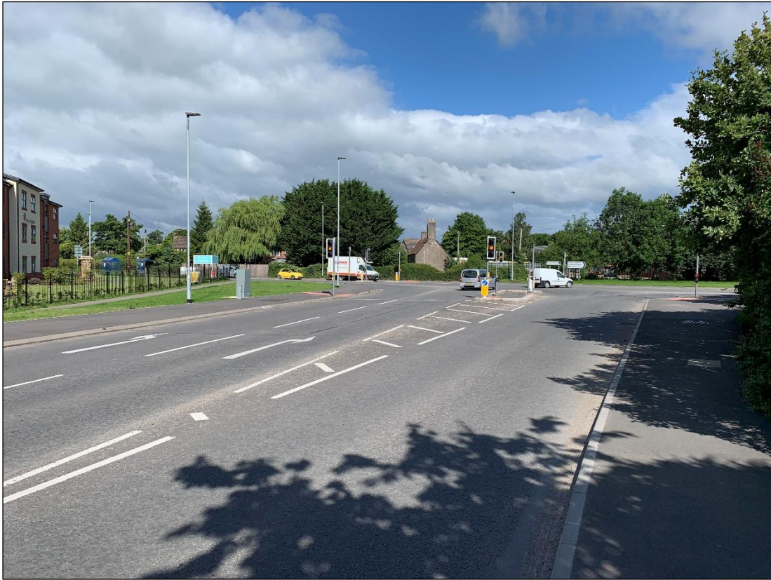
Photograph 3.5: View to the north along Windsor Drive to the A361 London Road/Windsor Drive Signal Controlled Junction
