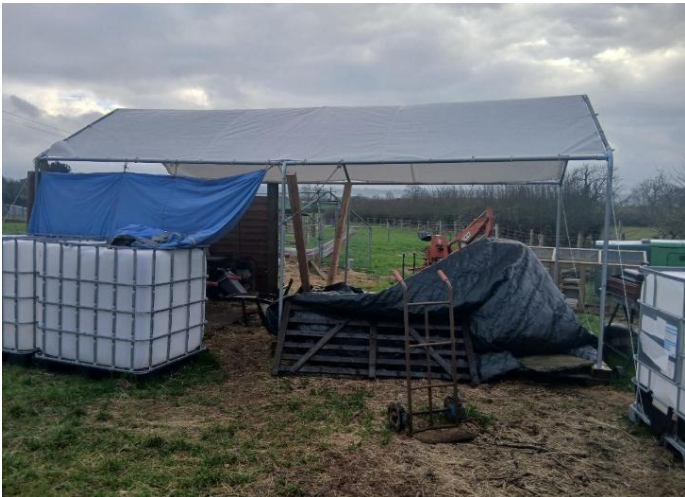
Open metal framed building to be removed
