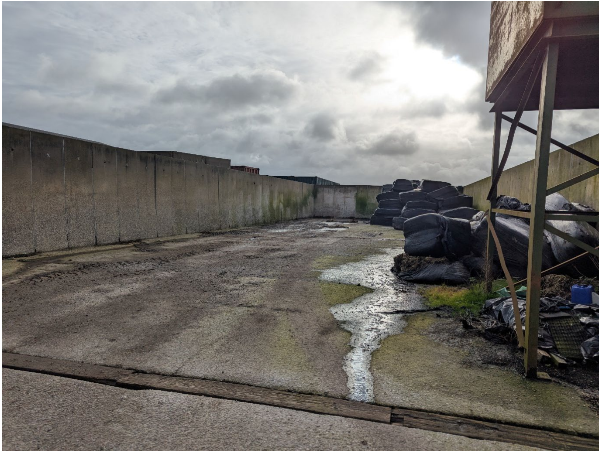
FIGURE 7: EXISTING SILAGE CLAMPS
