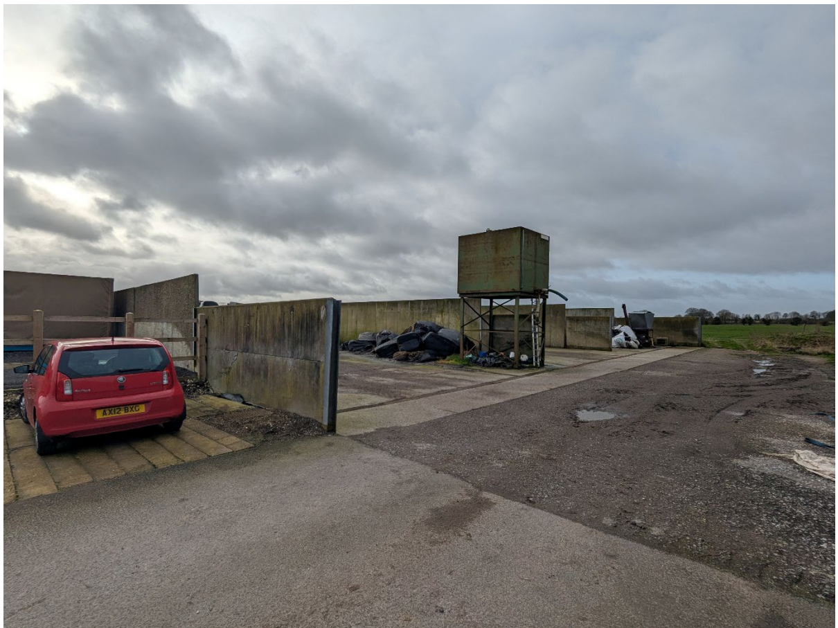
FIGURE 6: EXISTING SILAGE CLAMPS
