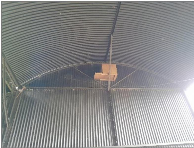
Photo 2. Roof structure of the barn (B1) with owl box
