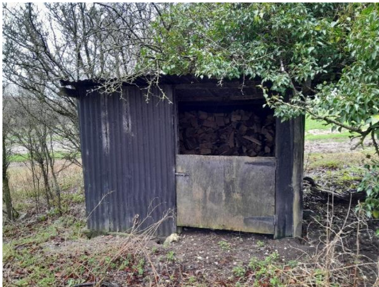
Photo 6. Metal storage shed (B3)
