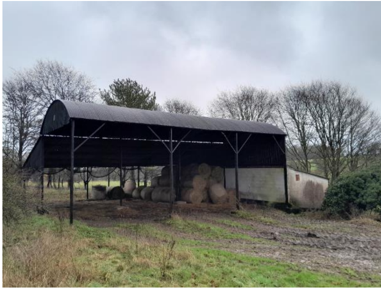
Photo 1. Northern and western elevation of the barn (B1)
