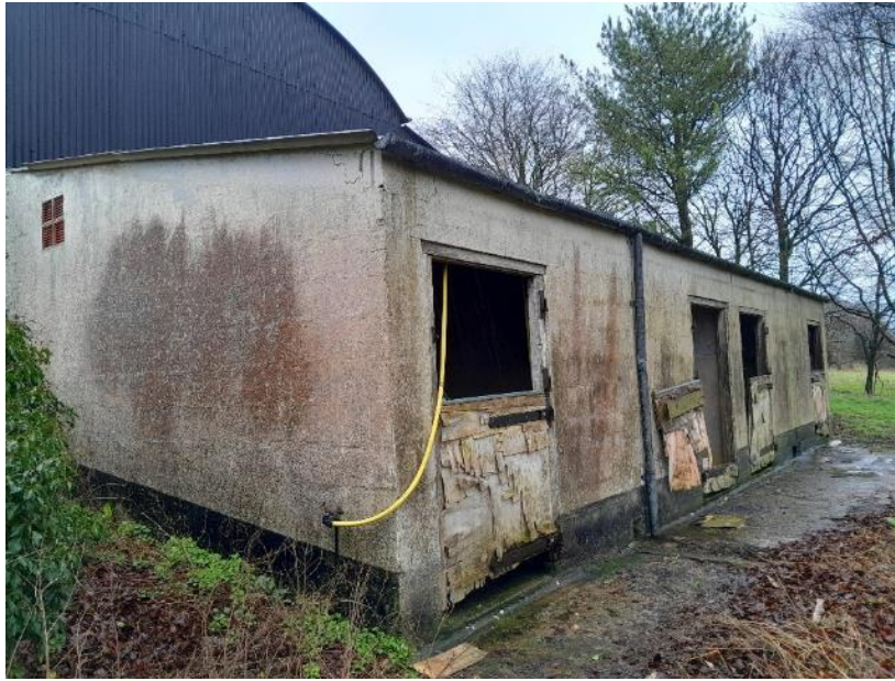
Photo 3. Southern and western elevations of the building (B2)
