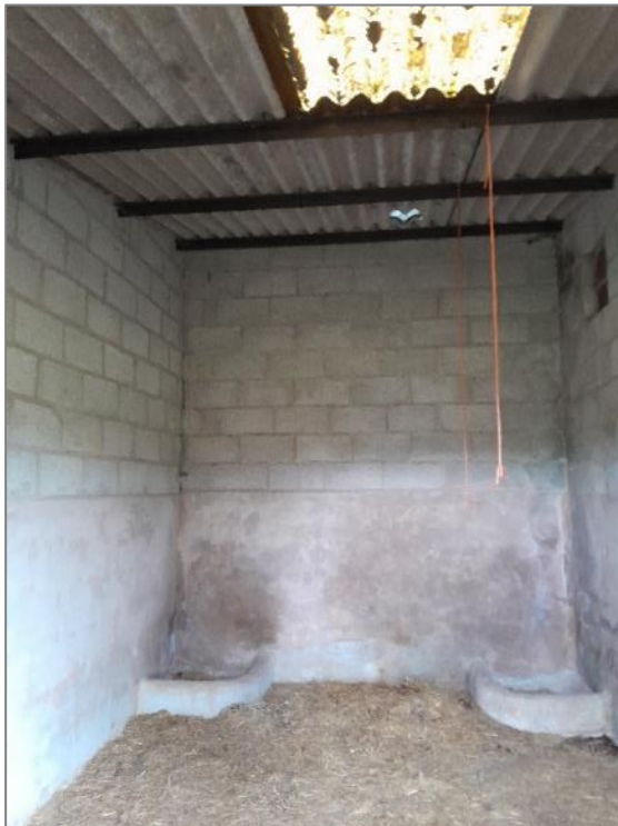
Photo 4. Internal compartment of building (B2)
