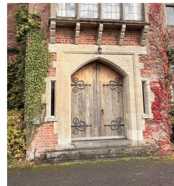
Site Picture of External Heritage door
