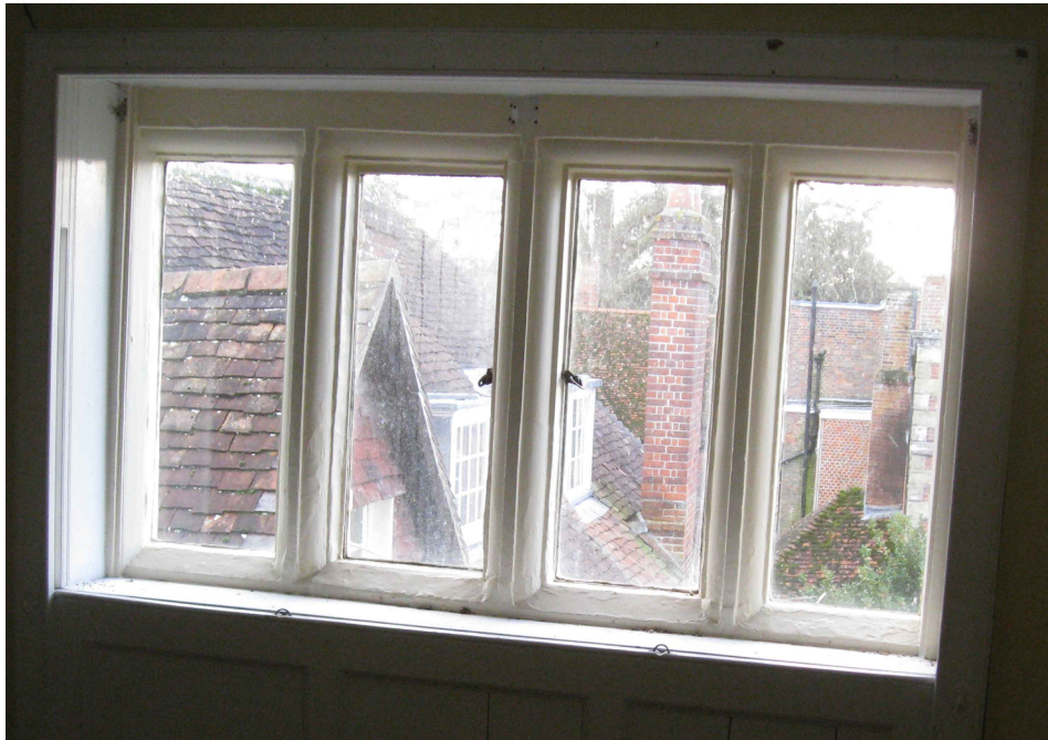
Photo from interior
