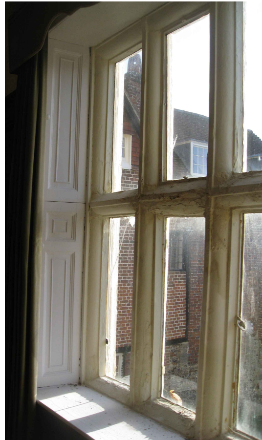
Image showing typical degradation of stone.
