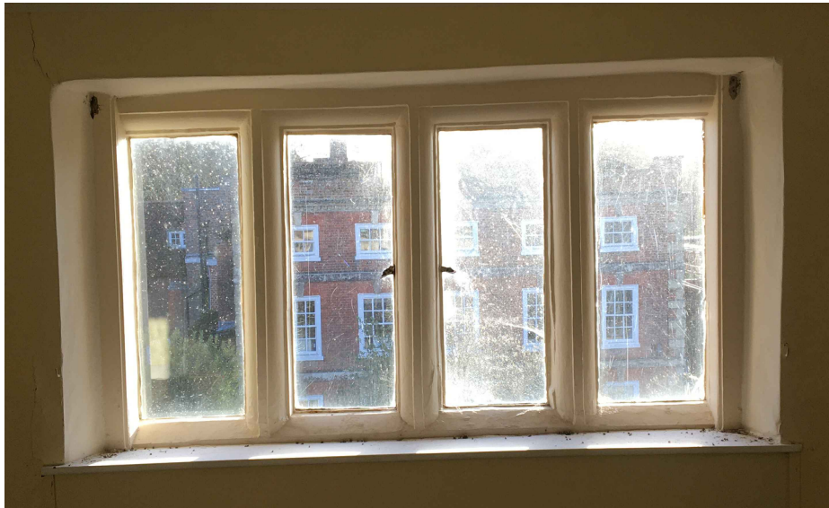
Photo from interior
