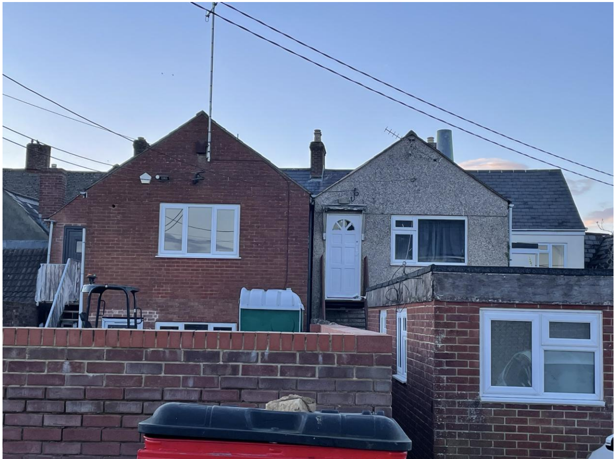
View from the rear access lane showing (L-R) rear glimpse of 118, 117 in the middle, and 116's rear residential access
