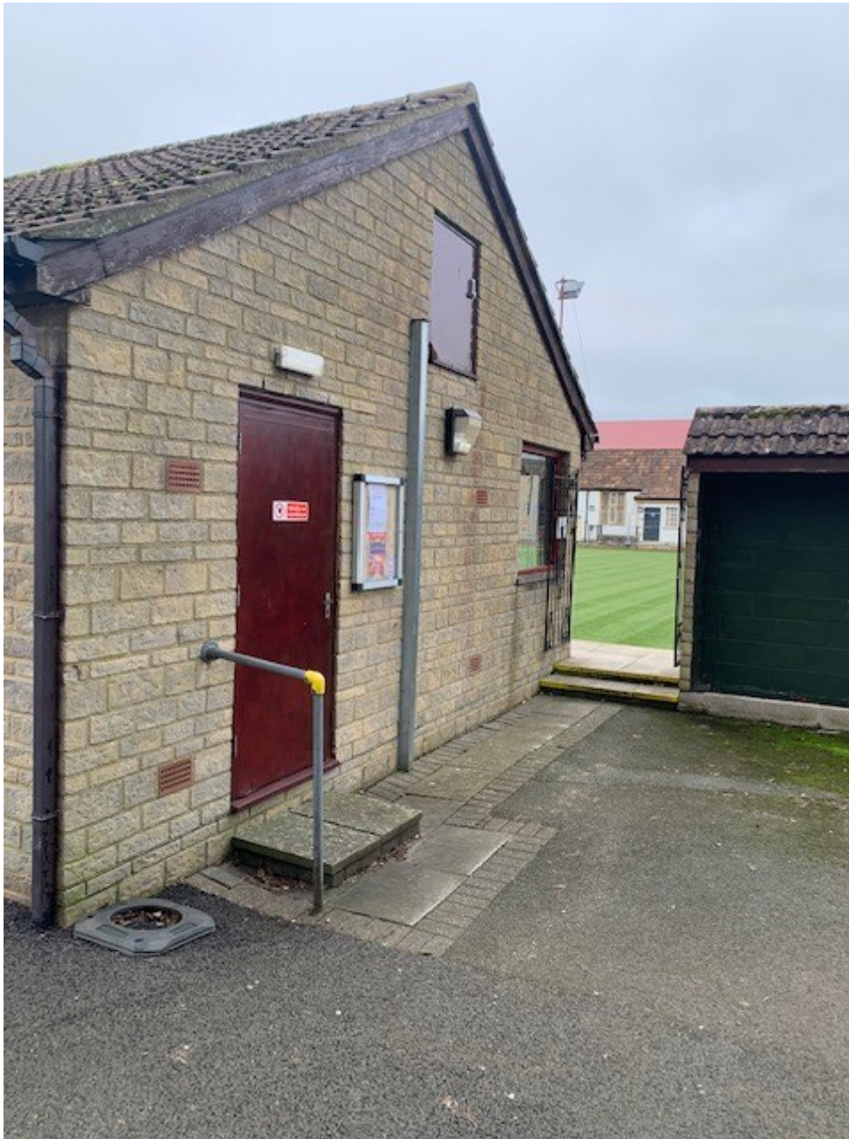
Western elevation of Club House
