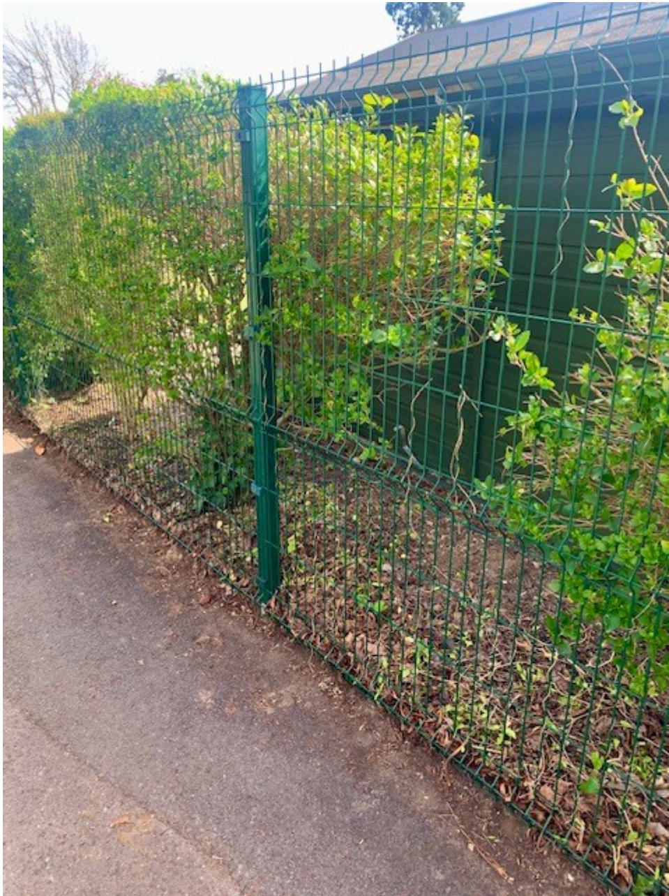
Existing fence (part) to northern boundary
