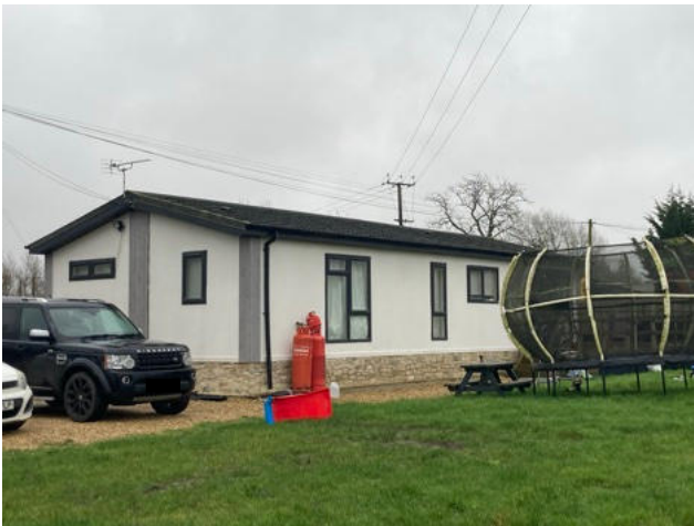
Image 7: North and western aspects of the building.
