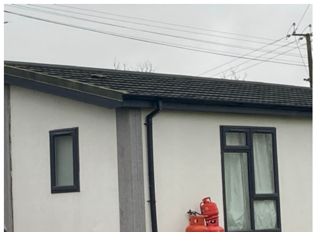
Image 12: Tightly fitted roof tiles.
