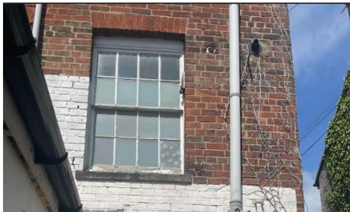
Figure 1: View of exterior window from courtyard.
