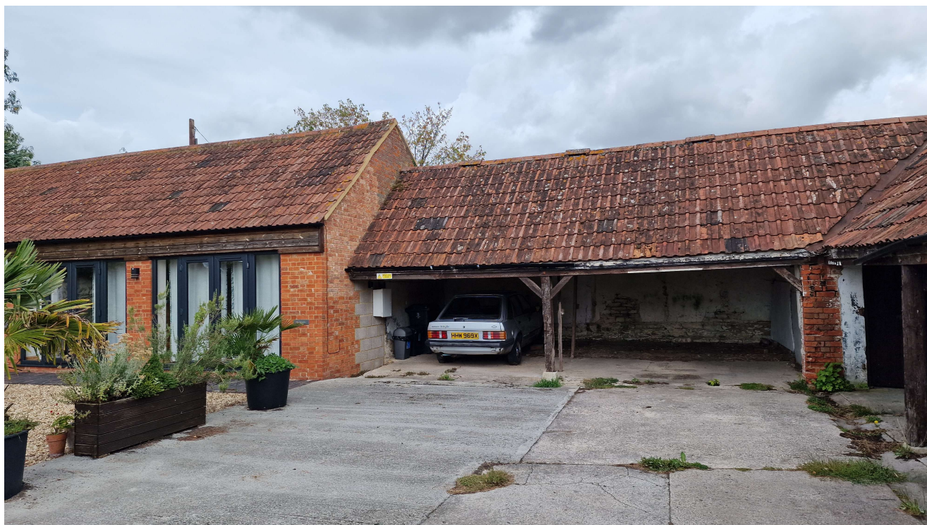
Right side of barn (south facing) showing existing open garaging to be converted to extend unit 1.
