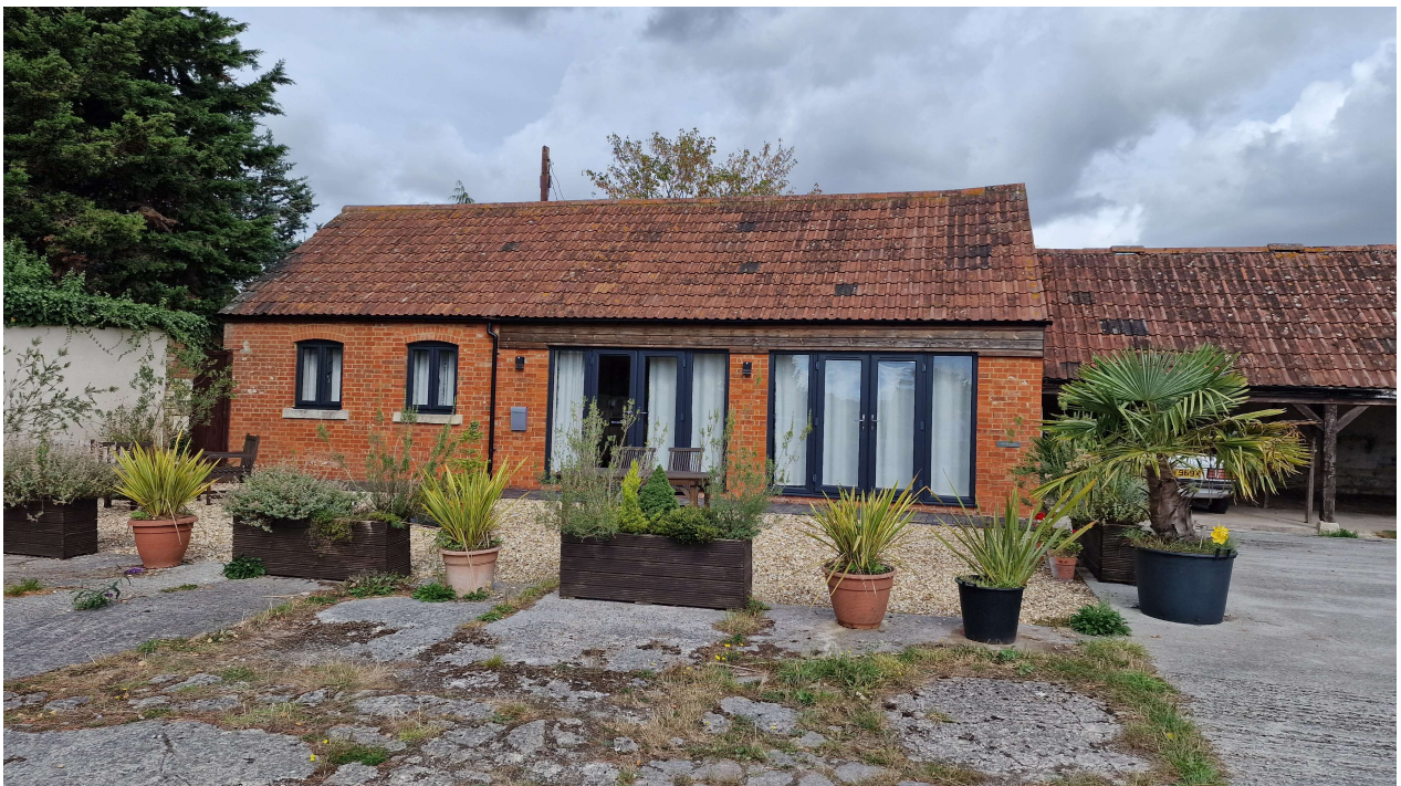
Existing frontage or south facing elevation of unit | converted earlier and in use.
