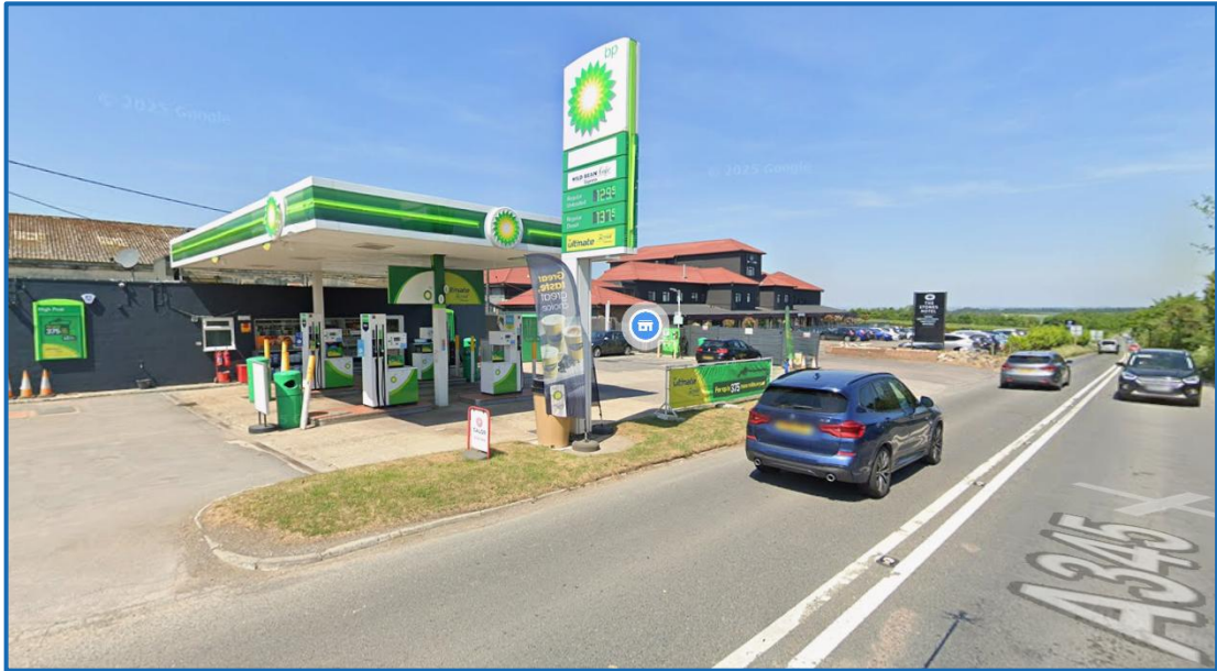
Figure 12: Existing Lighting of the BP Fuel Station on A345
