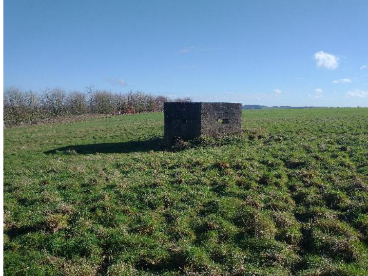
Figure 11: External aspect of the pillbox.
