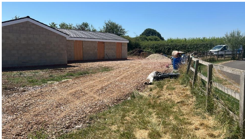
Existing Stable Block
