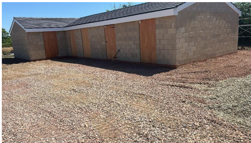
Existing Stable Block
