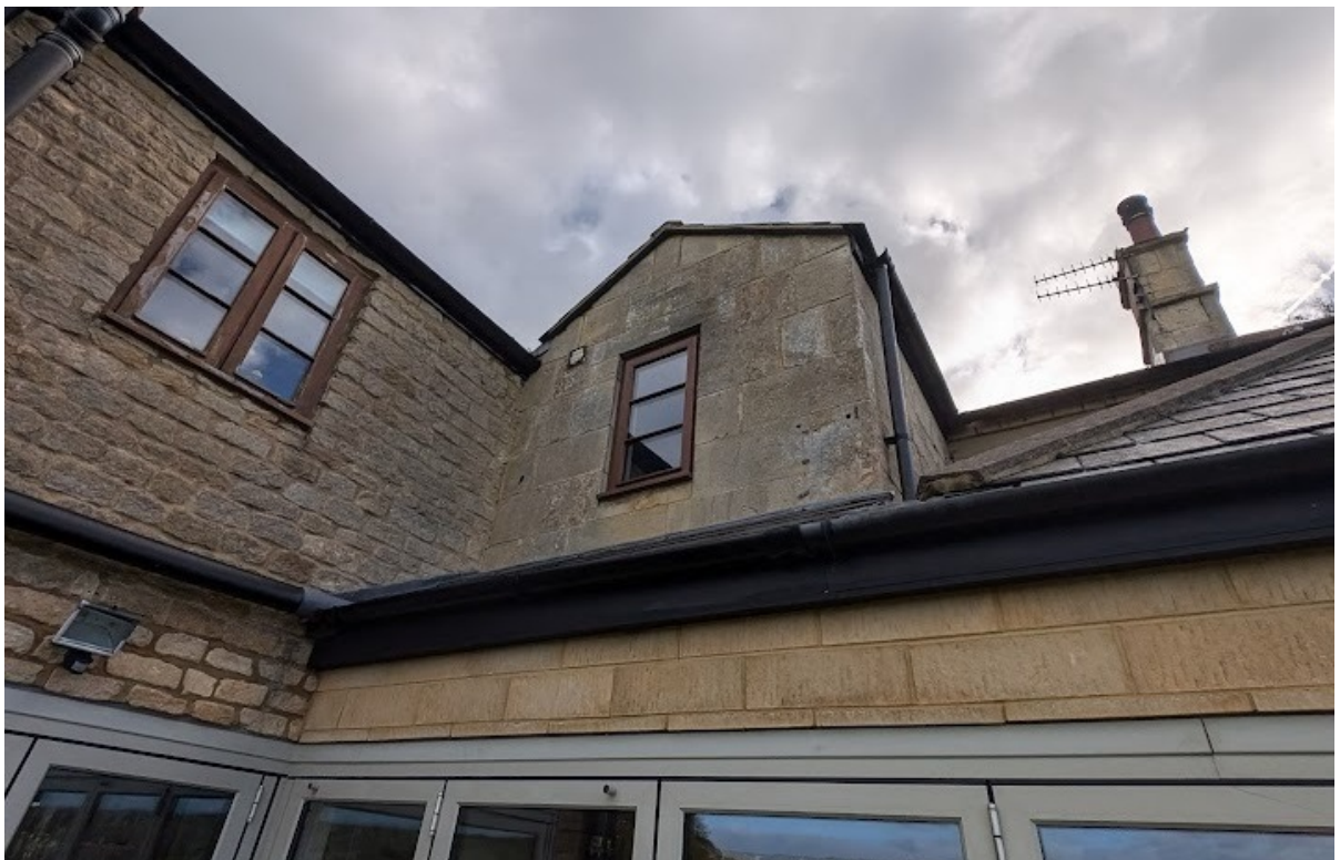
View of rear extension to be enlarged with extension below
