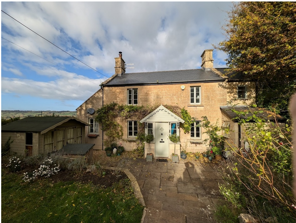
Front or south east facing elevation of 'Hillside', Quarry Hill, Box,
