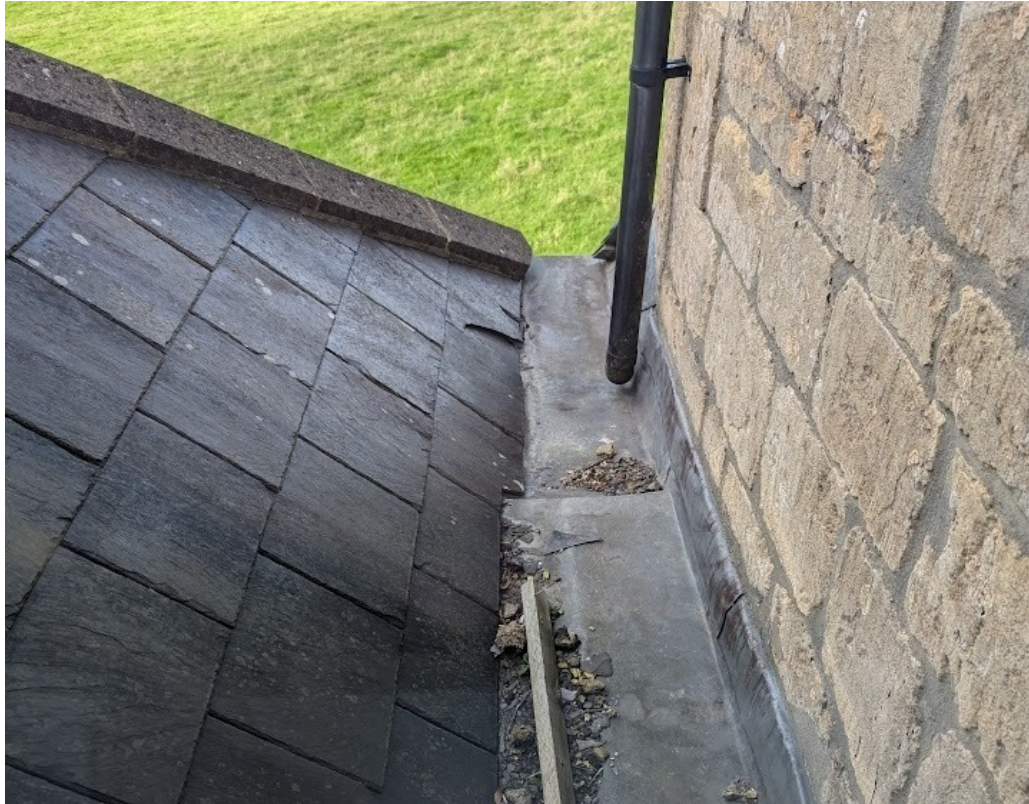
Rear hipped roof and valley gutter (to be removed and replace with flat roof detail as plans.
