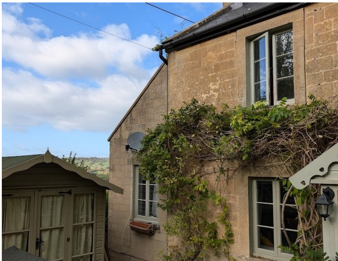
Close up front elevation of the property showing gable parapet to side extension (to be lowered).
