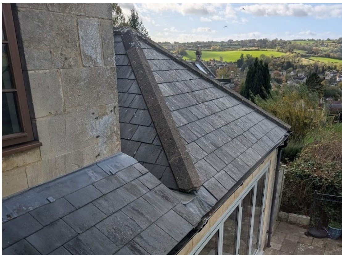
Rear hipped roof and valley intersection with en-suite addition.
