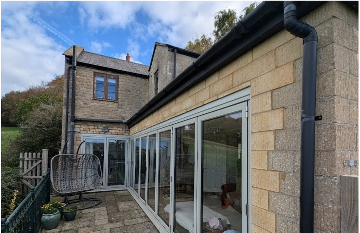
Rear elevation of property, smaller first floor extension to be enlarged in centre of picture.
