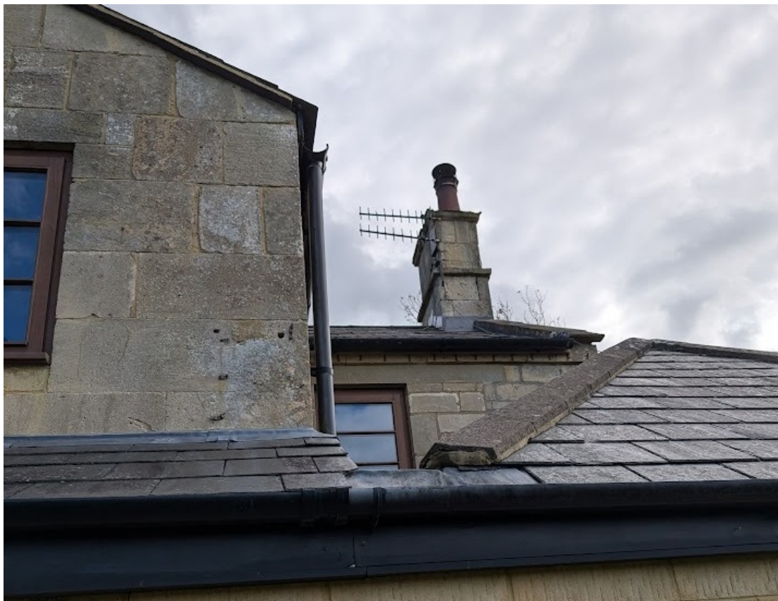
As above but showing hip roof and valley gutter abutment as well as small rear window to front bedroom
