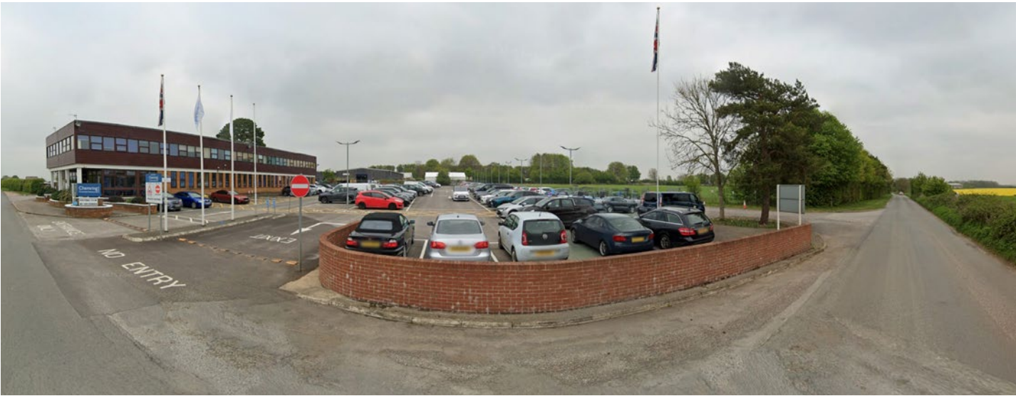
Panoramic View from the C292 of Chemring Countermeasures Existing Access
