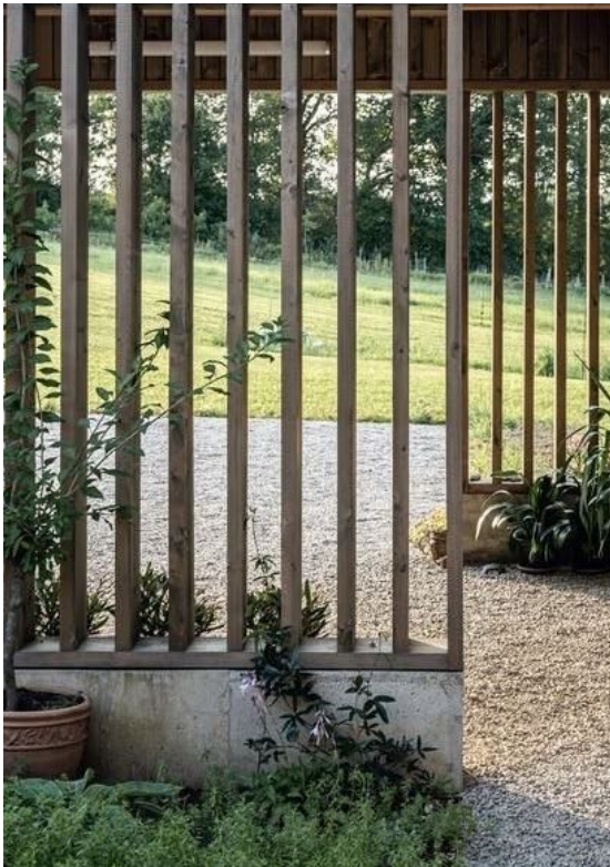
Timber slatted screen on wall Ref. 25-07-121
