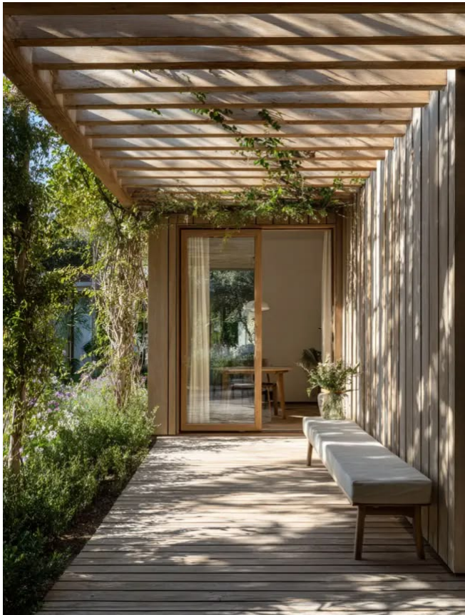
Timber pergola structure resting on garden wall Ref. 25-07-122
