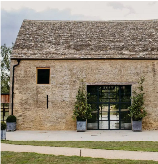
Crittall glazing within an existing opening Ref. 25-07-120
