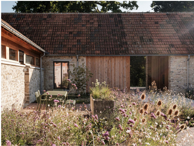
Timber infill cladding to existing door openings Ref. 25-07-121
