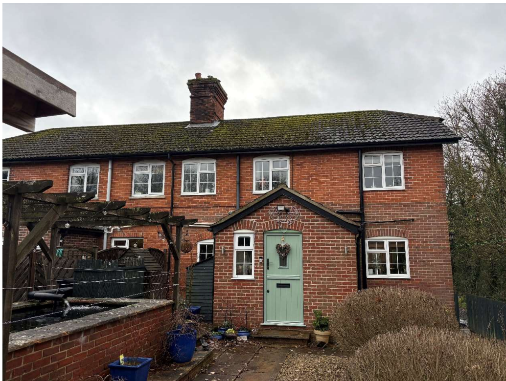
Figure 4 – Front (North) Elevation
