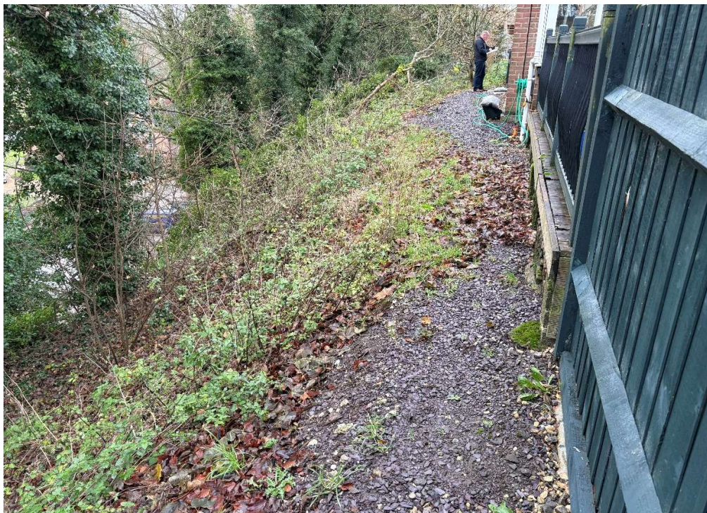
Figure 6 – Extent of slope / change in levels to side (West) of property
