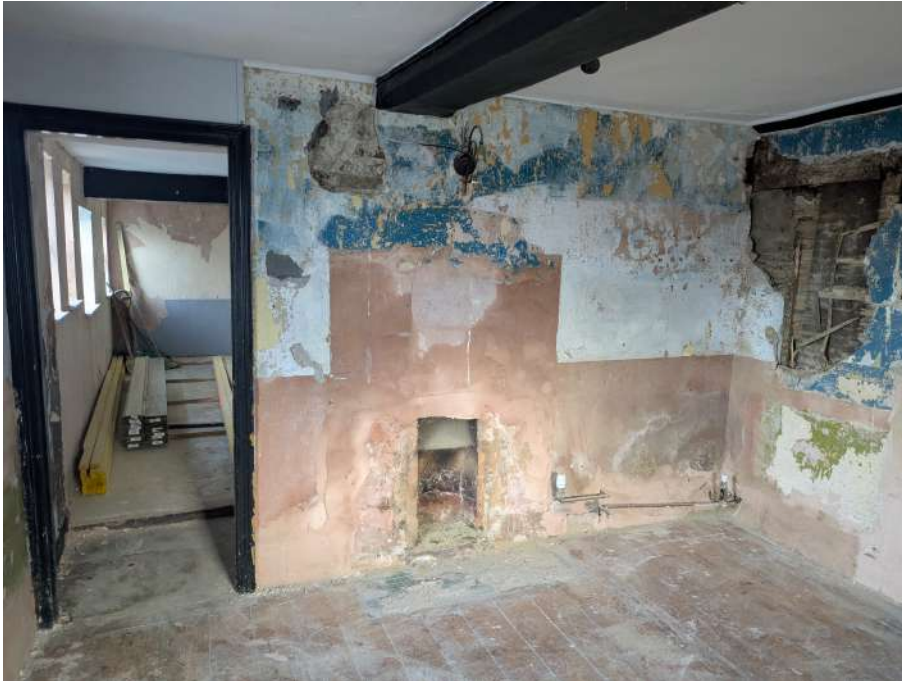
9. Chamfered beam and fireplace, private bar/pool room
