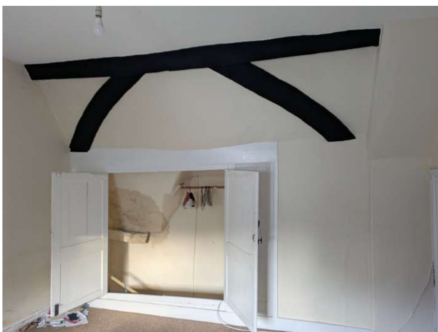
20. Wind bracing in C16 extension to hall, first floor
