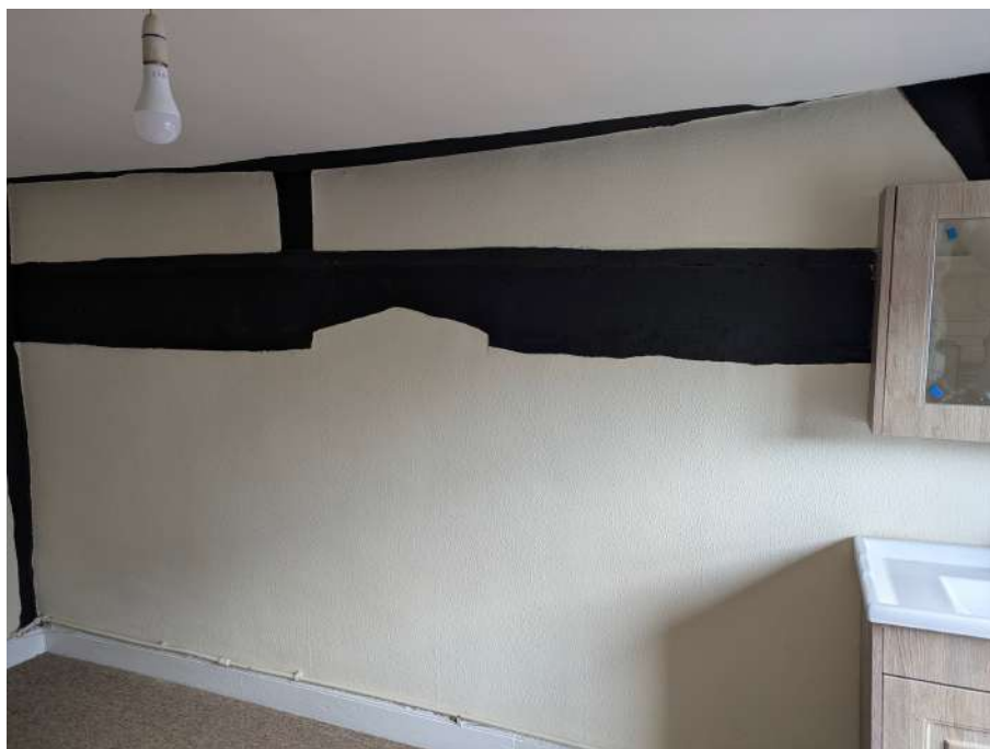
23. First floor; depressed Tudor arch door lintel.
