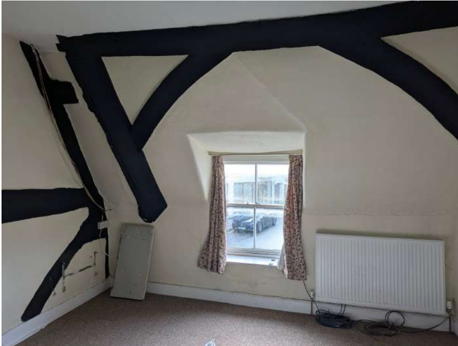
21. Windbracing and timber framing in C16 extension, first floor
