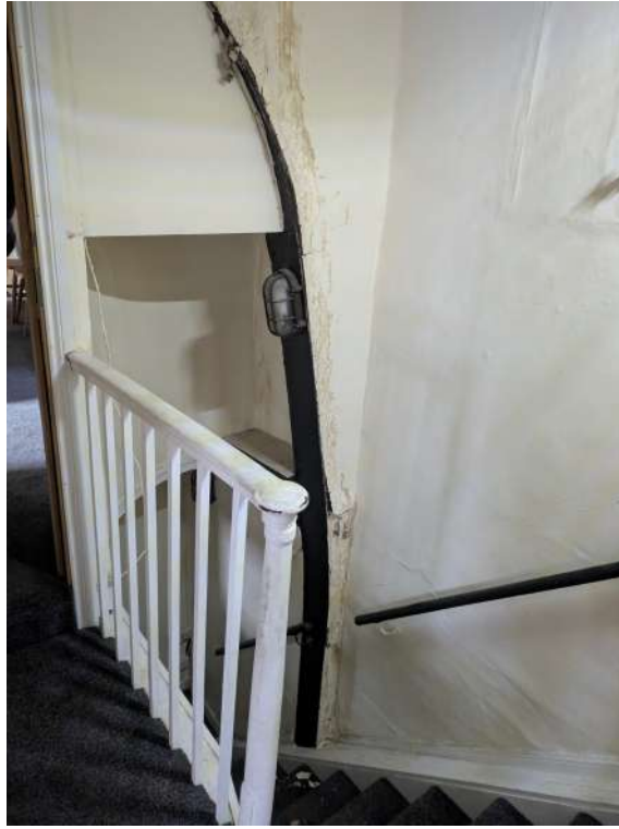
17. Base Cruck alongside staircase
