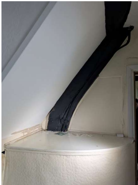
18. Base Cruck in corridor rising from staircase
