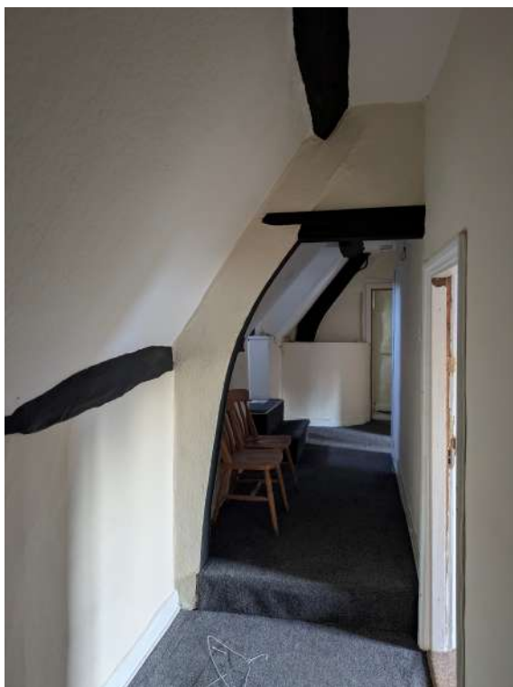
19. First floor corridor with base crucks
