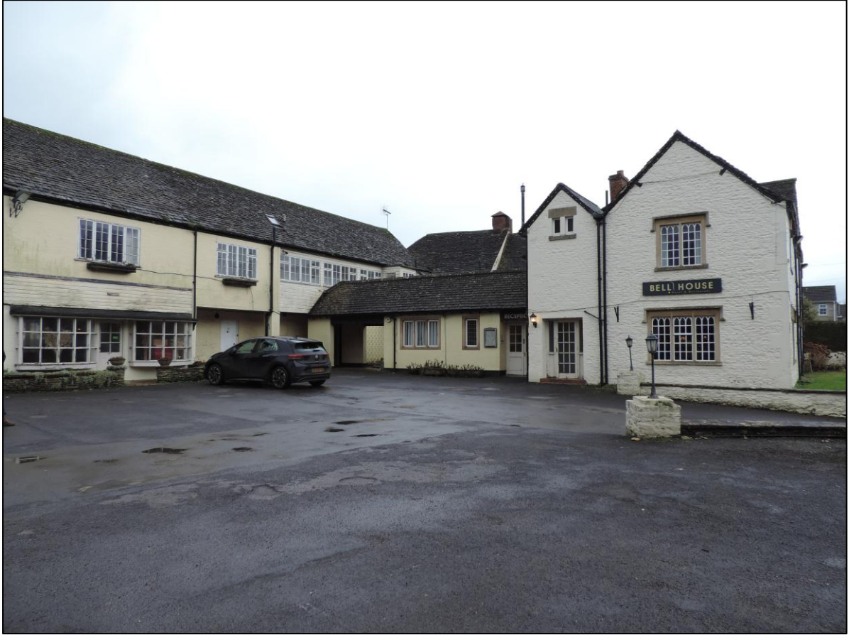
Photo 1 southwest facing view of The Bell House, from carpark. Historic core painted white.
