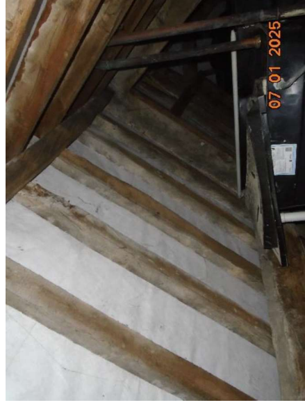
Photo 36: Internal of void 1.
