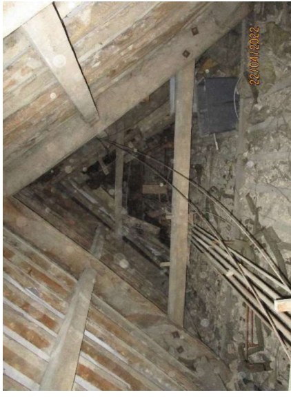
Photo 27: Internal of 'Void 2'.
