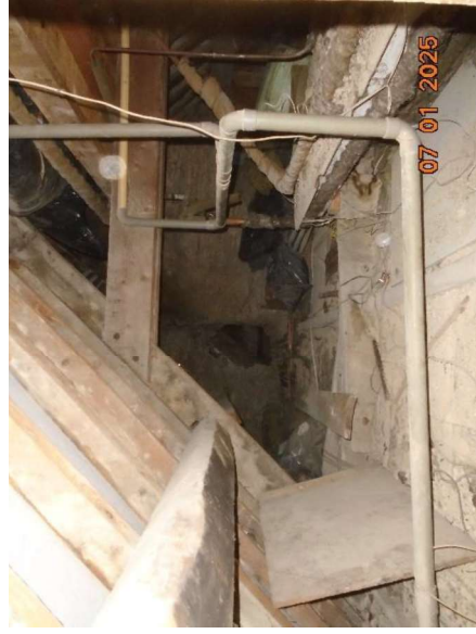
Photo 35: Internal of void 1.
