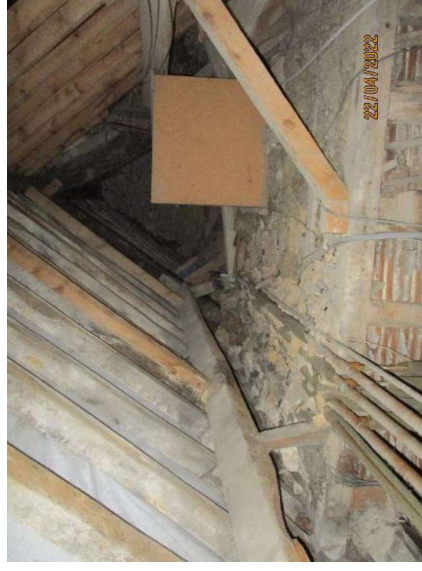
Photo 30: Internal of 'Void 2'.
