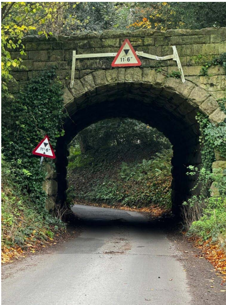
Approach to site from west showing restricted access at Mollys Bridge (Hatch House)
