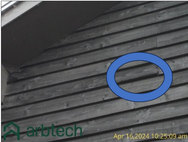
Figure 15- additional lifted boards on B1 southern elevation
