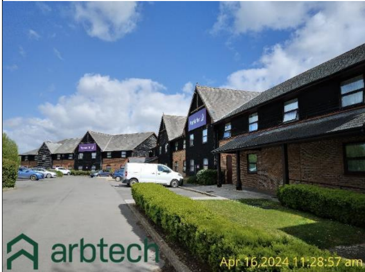
Figure 21- Overall view of B2- no proposed extension works on B2.
