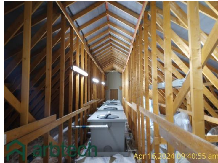
Figure 20 – Southern loft space of B1.
