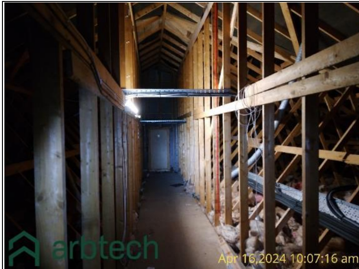
Figure 19- Northern loft space of B1
