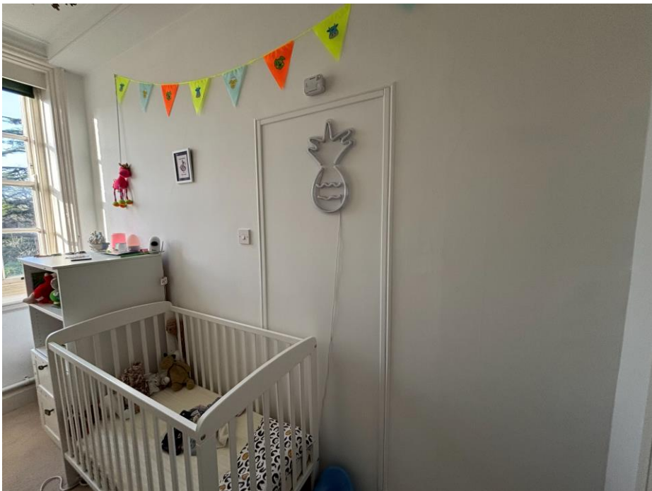
Fig.13: Bedroom 3 – interconnecting door blocked up
