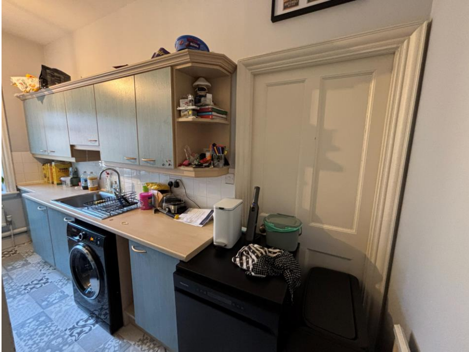
Fig.7: Modern eastern partition wall of Kitchen proposed for removal; 4-panel door to be salvaged for reuse within the flat
