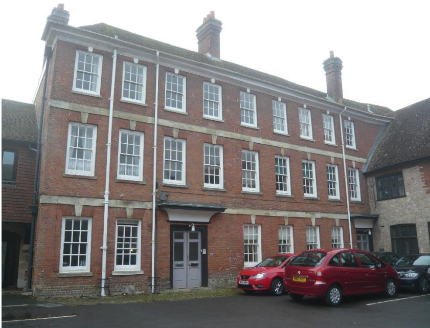
Fig.1: Front (north elevation) of South Block
