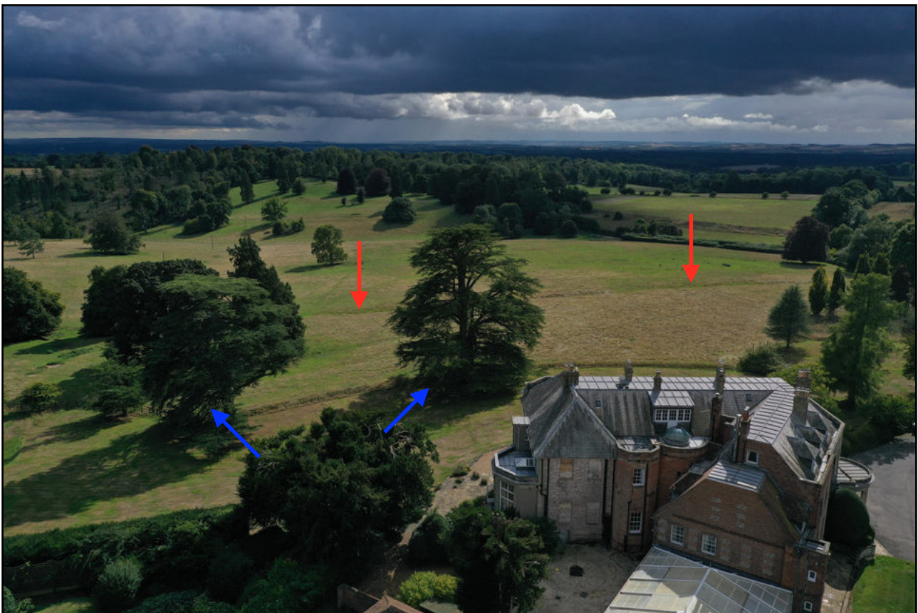
Figure 3.3.9: An aerial view is an effective way to illustrate the sunk fence (red arrows), as it is almost indiscernible in the landscape from close to the house at ground level (see figure 3.5.4, below). Two of the three cedars are visible to the left of the house (blue arrows). The tree on the right is likely to have been planted by Sir Sidney Meadows. The other c1760s cedar is just out of shot on the left. (Photo: Marie-Louise Agius).
