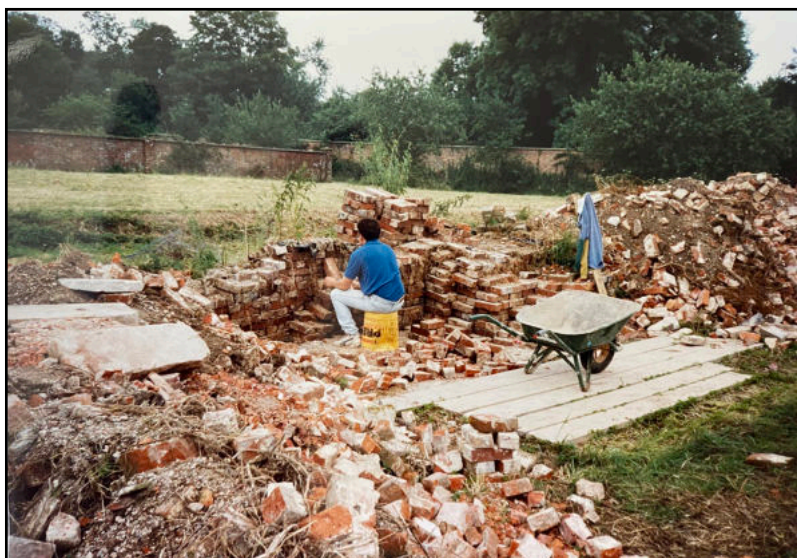
Figure 3.9.2: Rebuilding the walls of the kitchen garden in 1992. This is the south wall. The internal central wall can be seen in the background.
