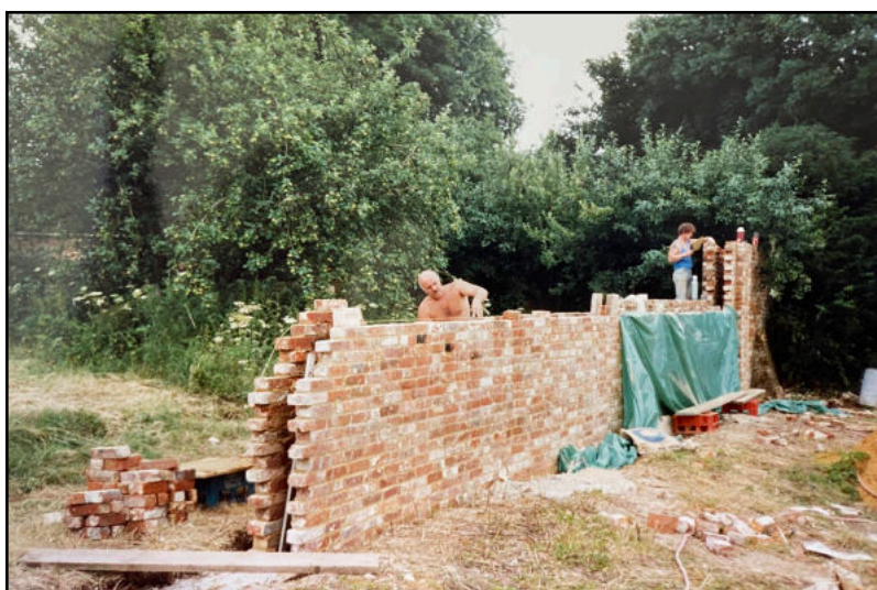
Figure 3.9.3: Rebuilding the walls of the kitchen garden in 1992. This is also the south wall close to the south-eastern corner.
