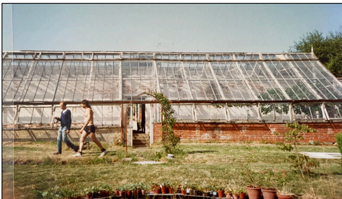
Figure 3.9.1: The old glasshouse and vinery in the walled kitchen garden, just before it was rebuilt in 1992. Note the small patches in the brickwork of the vinery on the right. These were blocked up holes through which the vines would originally have been grown. They were planted on the outside and trained through the holes. The different colours of brick work suggest this range of glass was built in two different phases.
