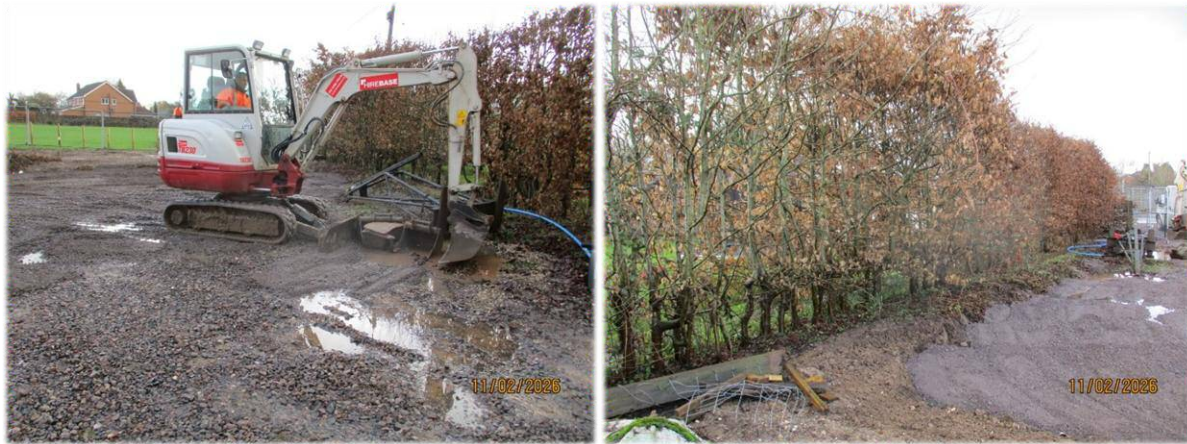
Southern boundary of the development plot with retained garden hornbeam hedge
