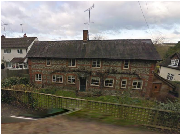
Hillside, South Street
