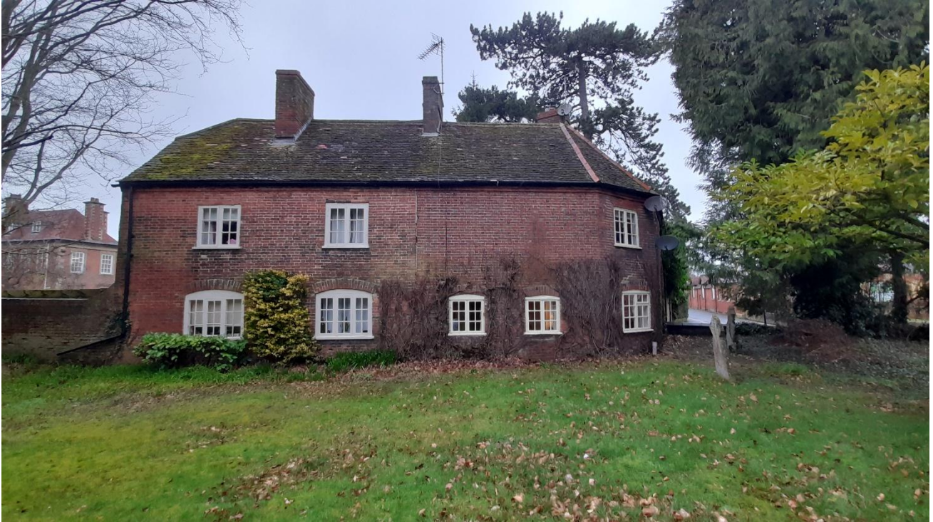
Photograph 4: The principal, east-facing elevation, seen from St Mary's churchyard and demonstrating the lack of invisibility with the proposed flue.
