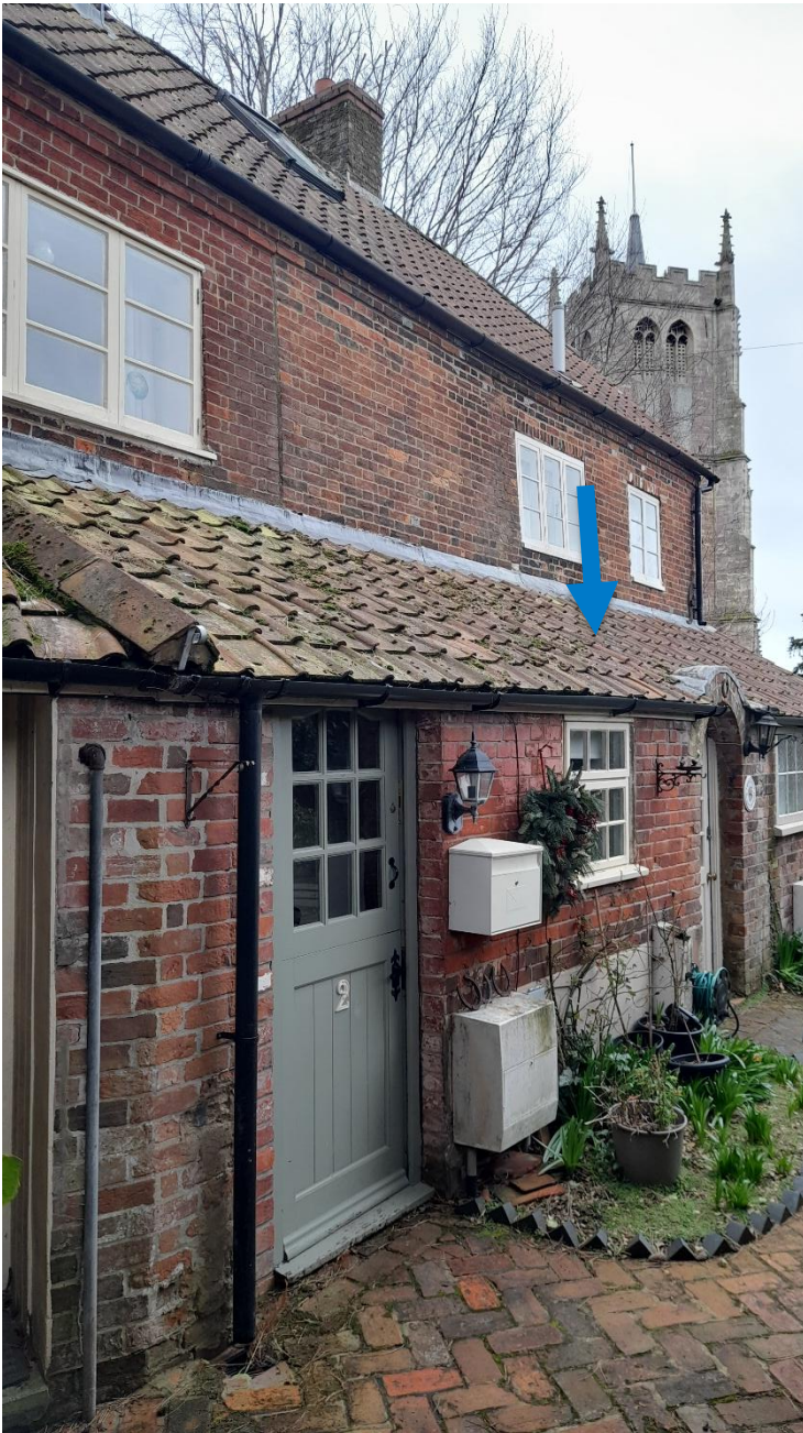
Photograph 1: The western elevation of Nos 2 & 3 St Mary's Cottages, with elements of the enclosed courtyard. The approximate location of the proposed flue is shown (in blue), with the 20 th century pantiles, neighbour's soil pipe above, and adjacent Grade I listed church shown. The alterations to the doorway to No. 3 are also visible.
