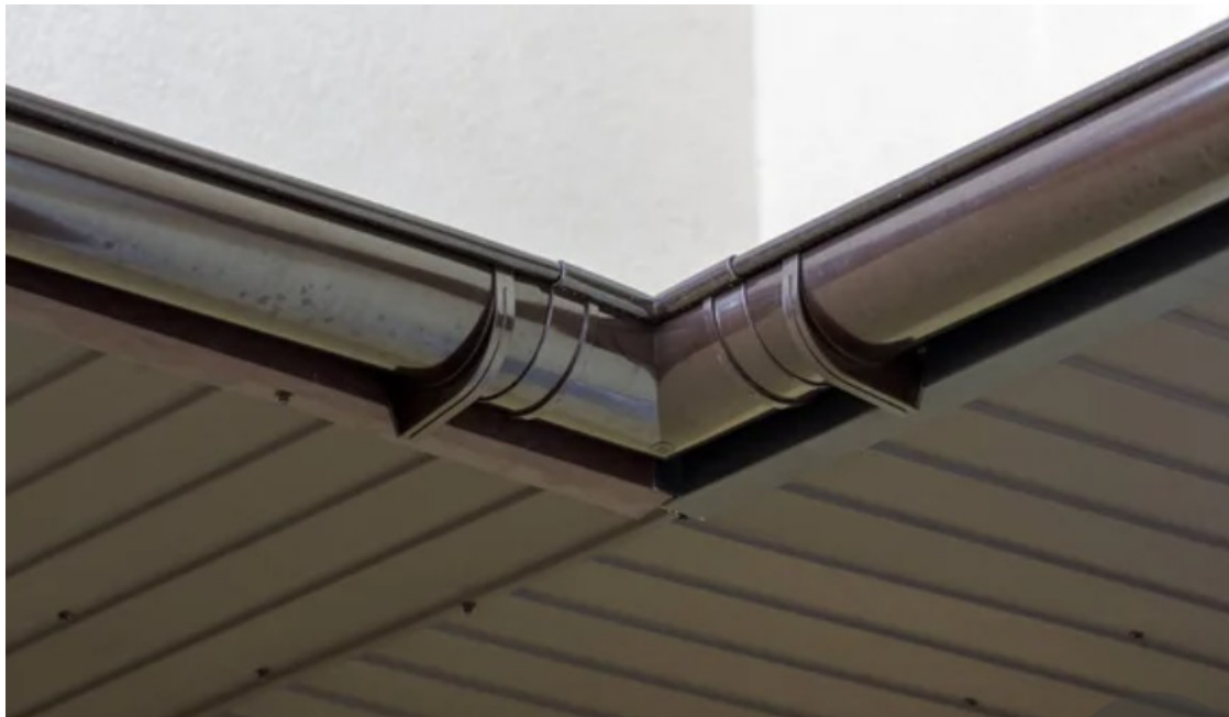
Bronze roof edge/ rainwater goods
