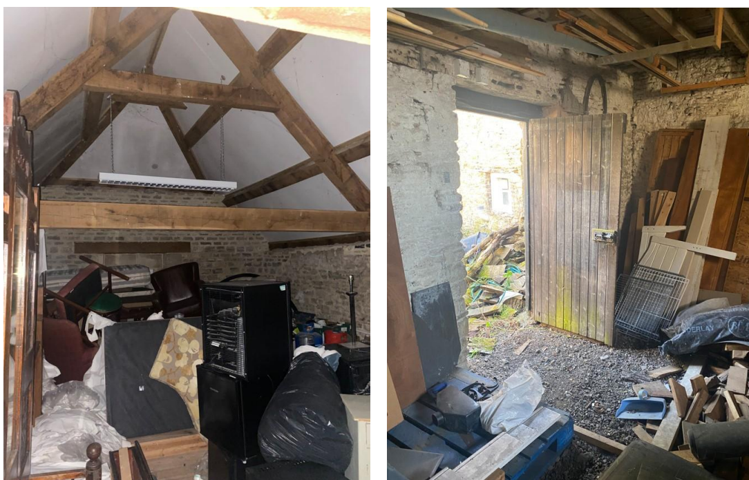
Interior of barn at first floor level (left); interior of adjoining single storey outbuilding (right)
