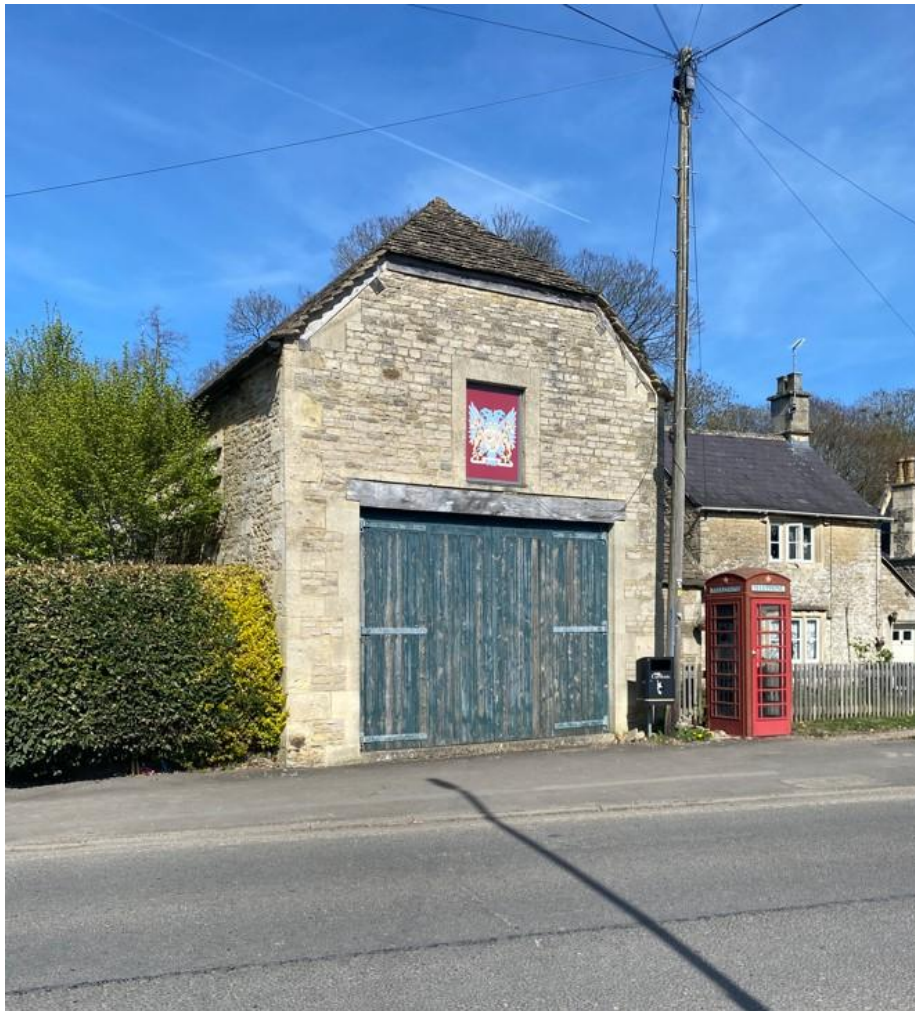
South elevation of the barn
