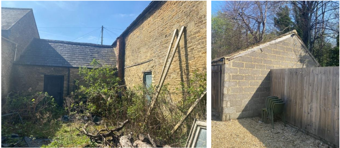
Rear elevations of barn and outbuilding (left); south elevation of storage barn (right)
