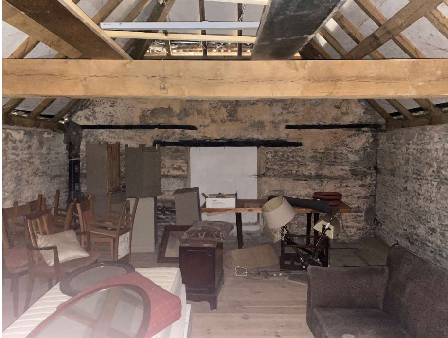
Plate 29 – View north through the first floor of the main range.
