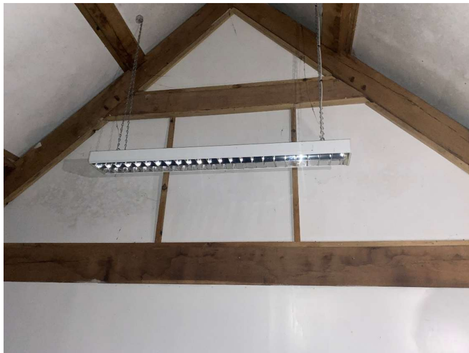
Plate 28 – Insulation boards installed to modern roof truss.
