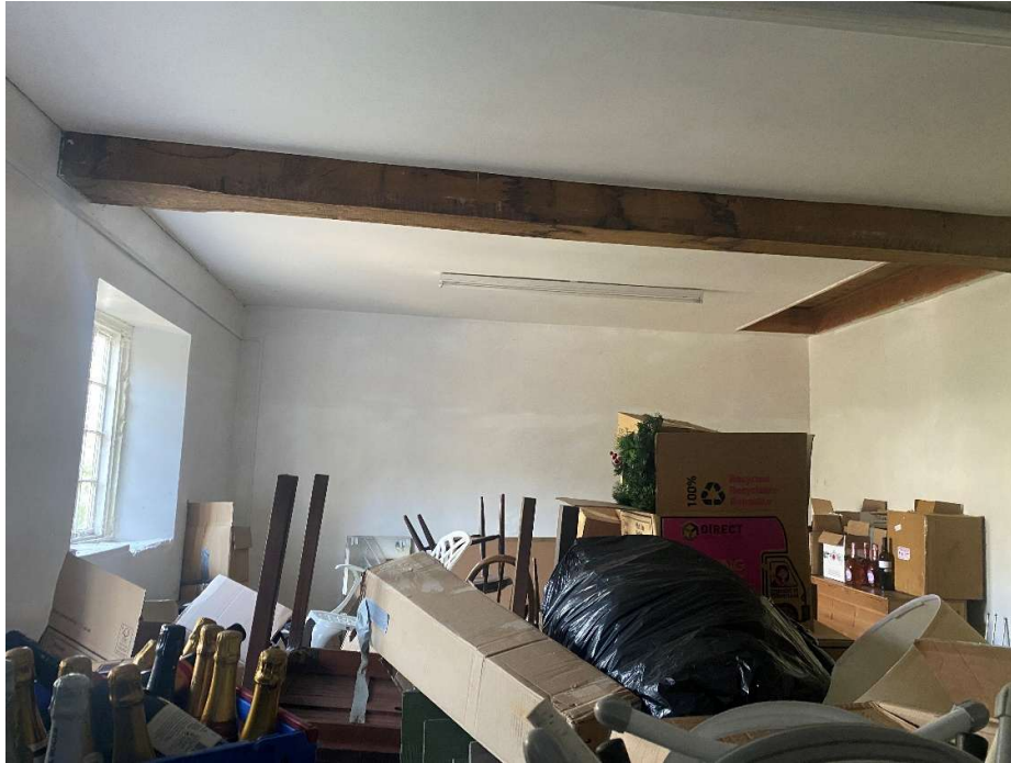
Plate 21 – View north through the ground floor of the main range showing modern ceiling and wall finishes.
