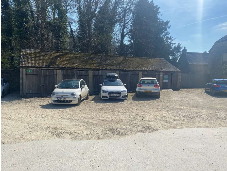
Plate 19 – West elevation of the modern garage / storage block which is to have cedar cladding applied to conceal the concrete blockwork piers and side elevations.
