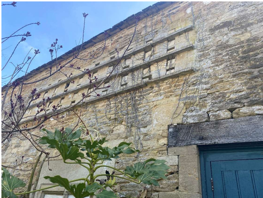
Plate 14 – Dove holes to the first floor of the west elevation.
