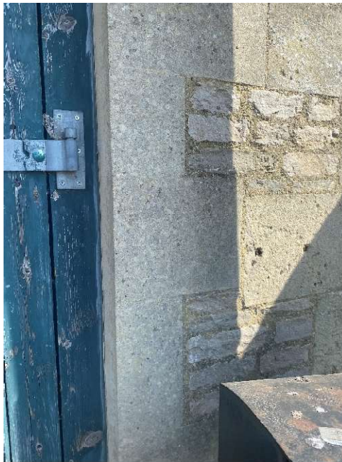
Plate 4 – Rebuilt stone quoin surround to double garage doors on the southwest elevation.
