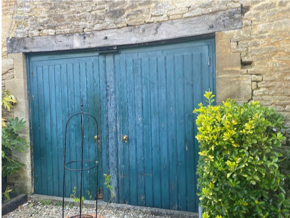
Plate 13 – Modern, double doors to the west elevation which are to be replaced with new entrance doors. Supporting central post and timber lintel to be retained.
