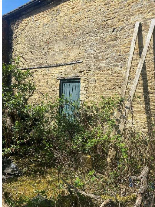
Plate 9 – Part southeast elevation of the main range with single boarded door where proposed extension is to be located.
