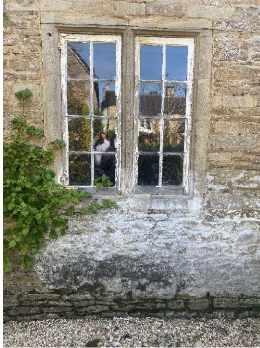
Plate 15 – Mullion window with timber casements to the ground floor of the west elevation.
