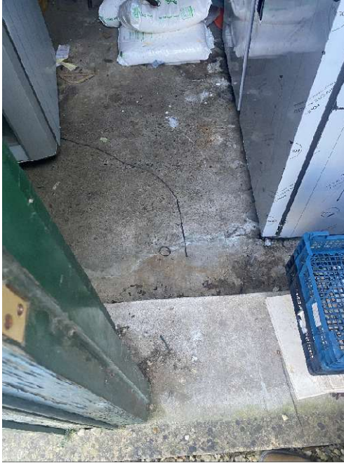
Plate 23 – Modern concrete floor to the main range of the outbuilding.
