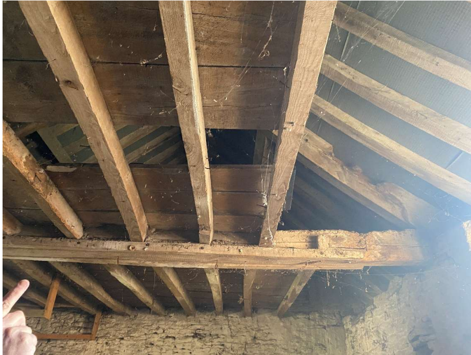
Plate 35 – Ceiling joists and beam to the east range.
