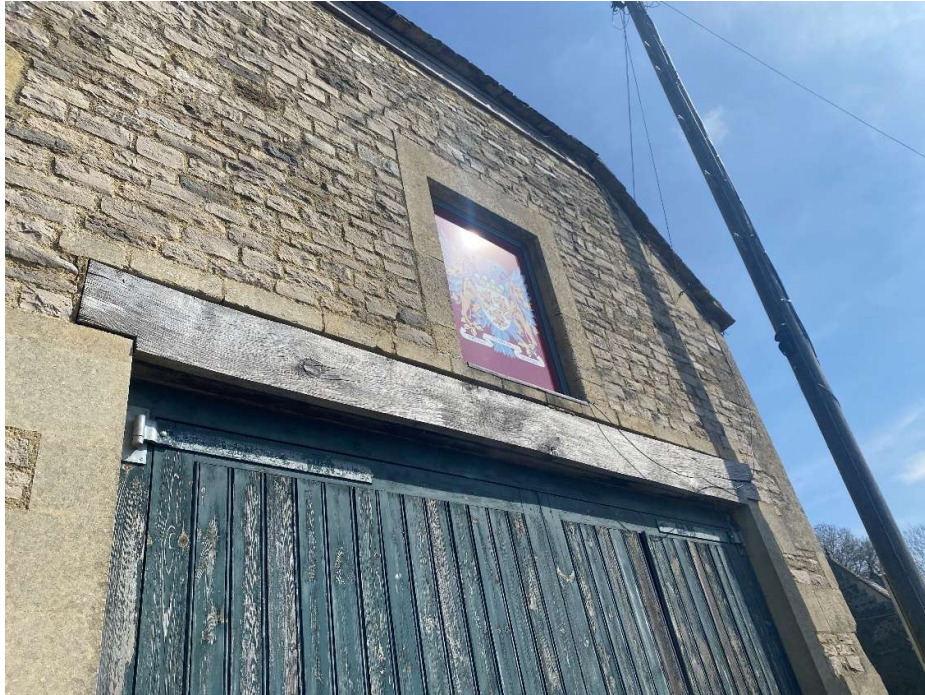
Plate 5 – Infilled opening to the first floor of the southwest elevation.
