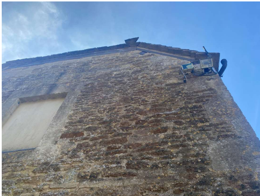
Plate 18 – Part north elevation showing blocked opening to the centre which is to have a new window inserted.
