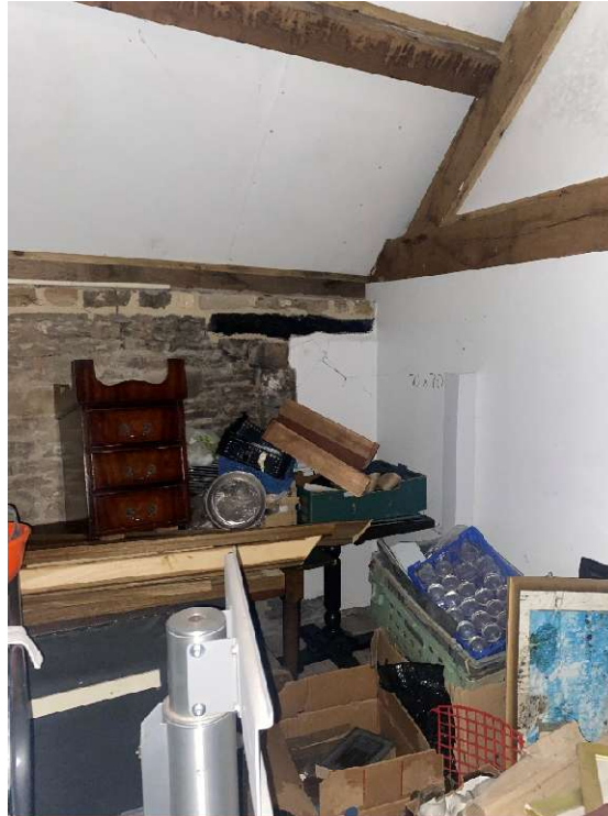
Plate 27 – View west towards the infilled opening to the first floor of the west elevation of the main range.
