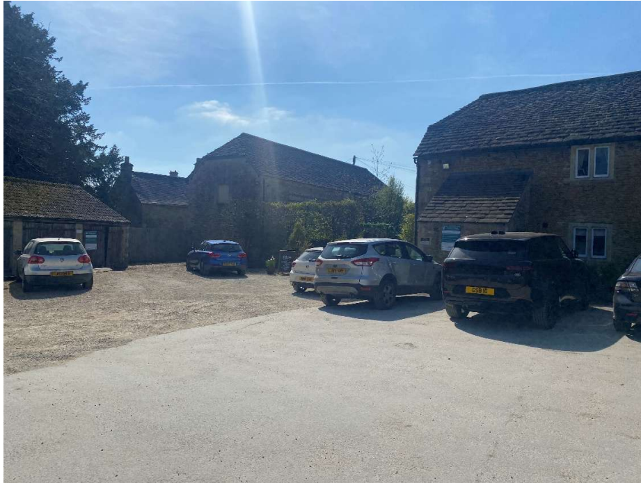
Plate 17 – The outbuilding range viewed from the car park area with part north and west elevations.
