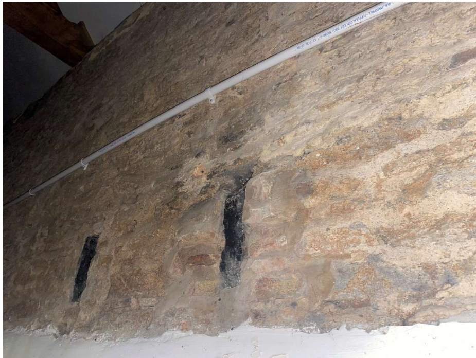
Plate 32 – Charred ends of earlier floor joists visible in the east wall.
