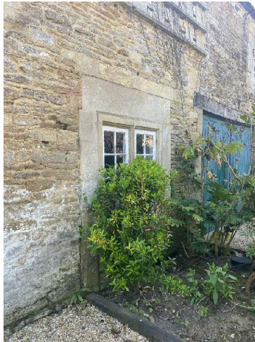
Plate 16 – Altered former door opening to the west elevation; now a window.
