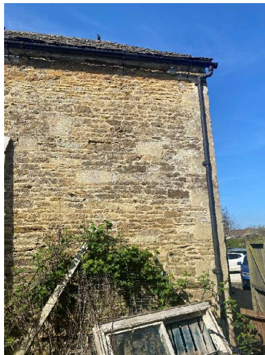
Plate 10 – north corner of the east elevation of the main range.
