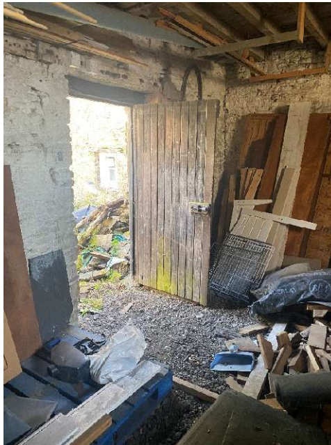
Plate 34 – Interior of the east range.
