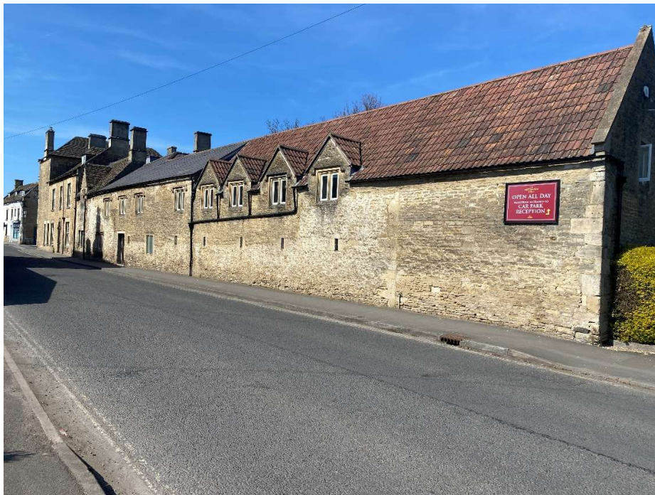
Plate 2 – Southwest elevation of the Methuen Arms Hotel viewed from South Place.
