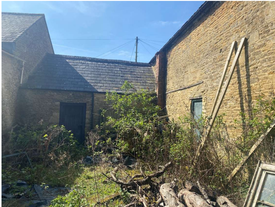
Plate 6 – Northeast elevation of the east range and part east elevation of the main range viewed from the rear courtyard area.
