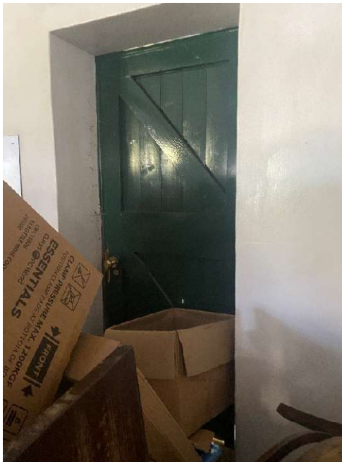
Plate 22 – Interior view of the boarded door to the east elevation of the main range.
