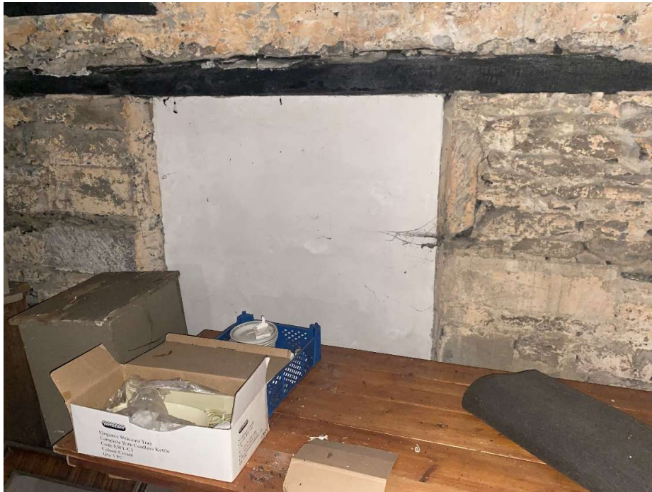
Plate 30 - Inflled opening to the north elevation where new window to match existing is to be inserted.
