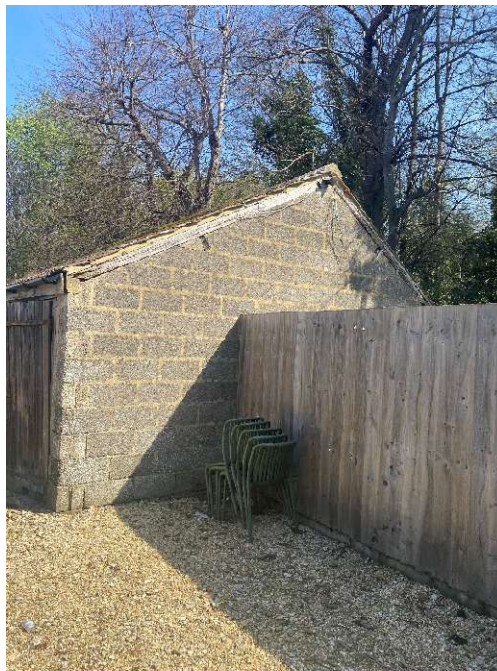
Plate 20 – South side elevation of the modern garage / storage block which is to be cedar clad.
