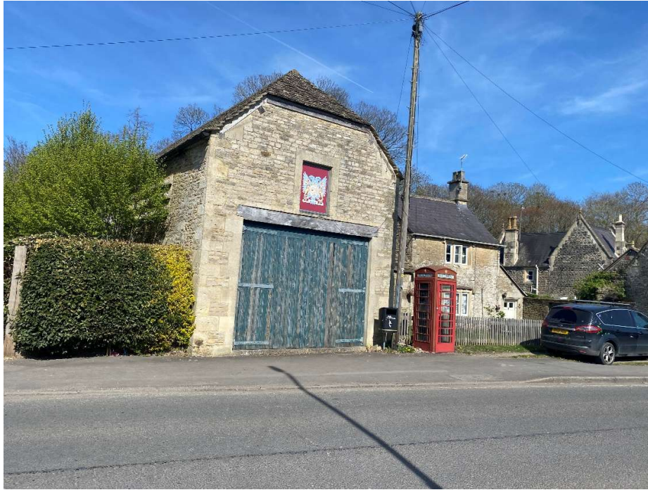
Plate 1 – Outbuilding viewed from South Place.
