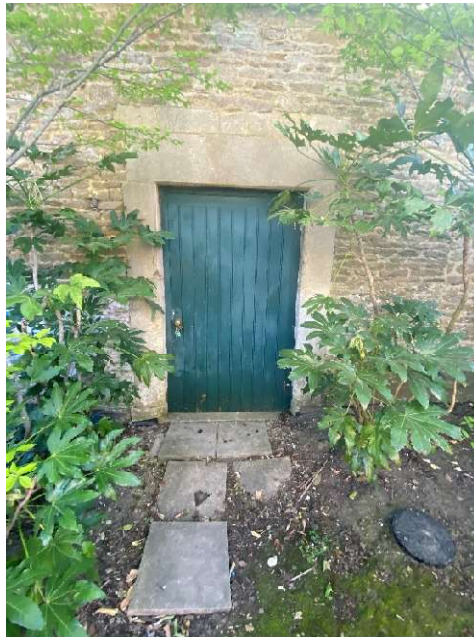
Plate 12 – Single boarded door to the west elevation which is to be retained.
