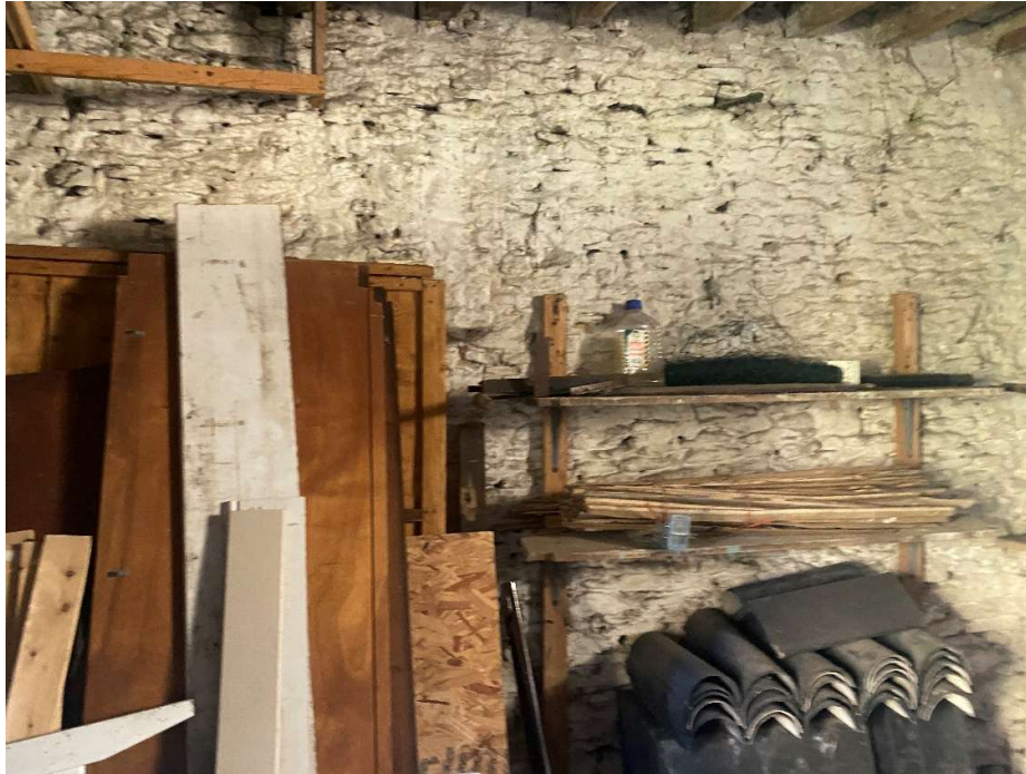
Plate 33 – Interior of the east range.
