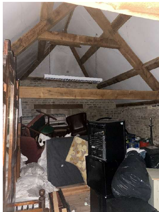
Plate 26 – View south through the first floor of the main range showing new roof timbers and insulation to the underside of the roof.
