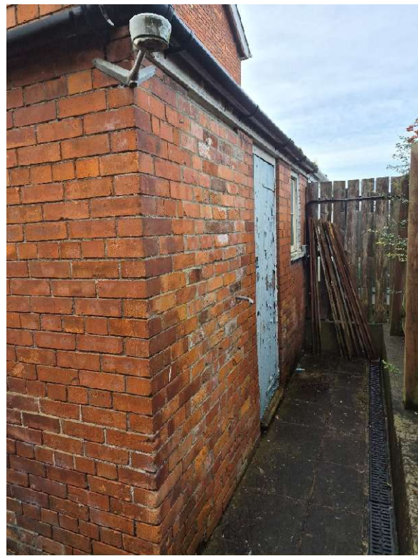
Lean-to section and boundary fence.
