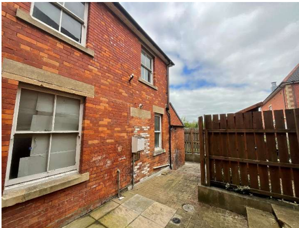
Rear Yard with Lean To Roof
