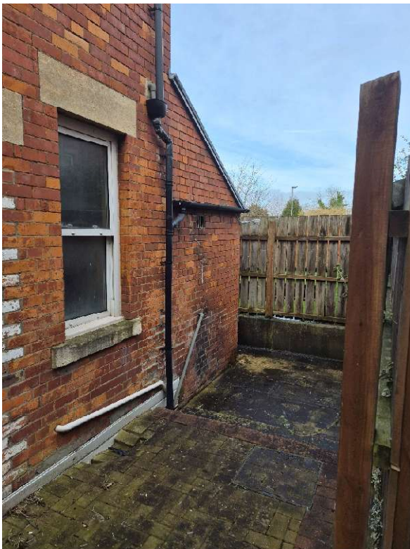
Rear yard – location of extension.
