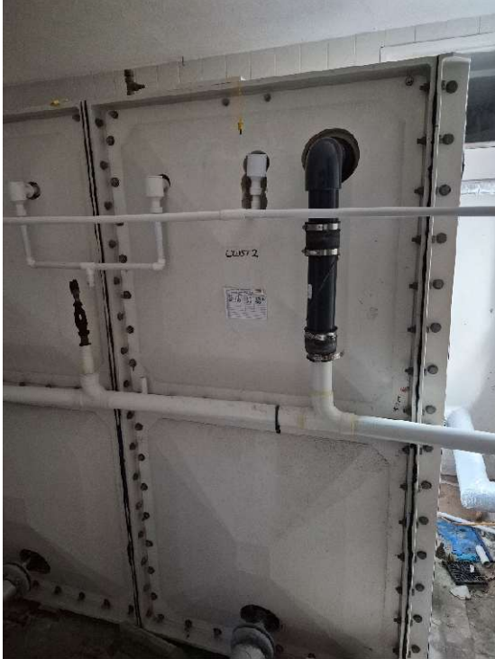
Existing large water storage tank
