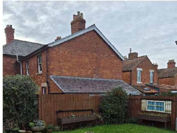
Rear gable and lean-to roof
